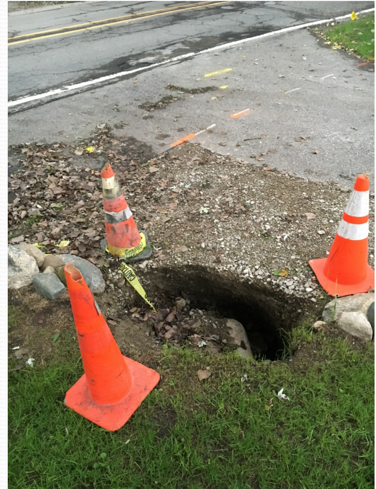
Emergency 3: Sinkhole over failed pipe
