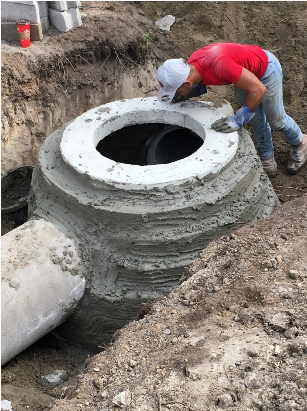
Emergency 1: Pipe and structure construction to replace failed pipe
