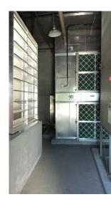
The system uses bacteria, which grow on an inert plastic medium, to oxidize the hydrogen sulfide. This biofilm removes 99 percent of the gas. The microbes convert the odorous compounds to oxygen and water—that are naturally occurring and not harmful to the environment. Odorous air is then pulled through ductwork to a blower that forces the air through the bacteria-covered media. Treated air is discharged at the top of the tower.
