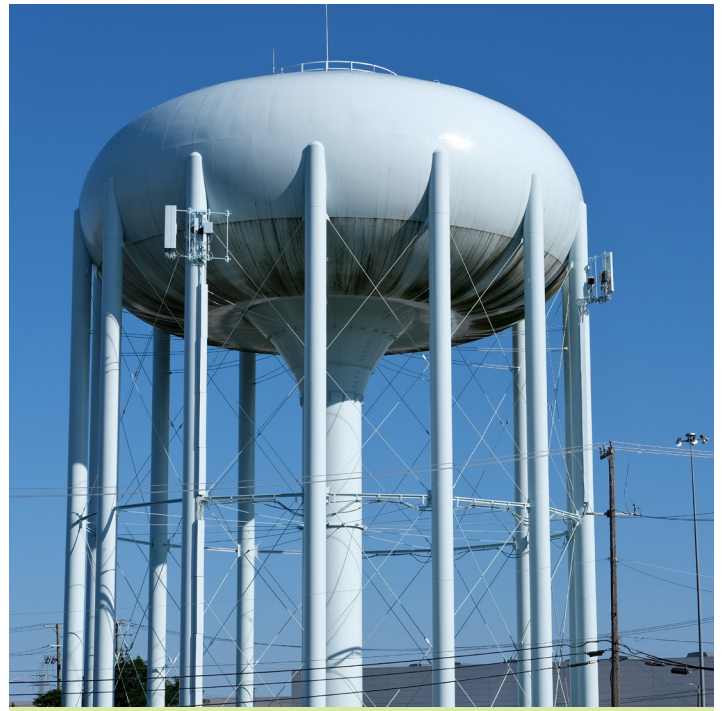
Water Tower, City of Pontiac
