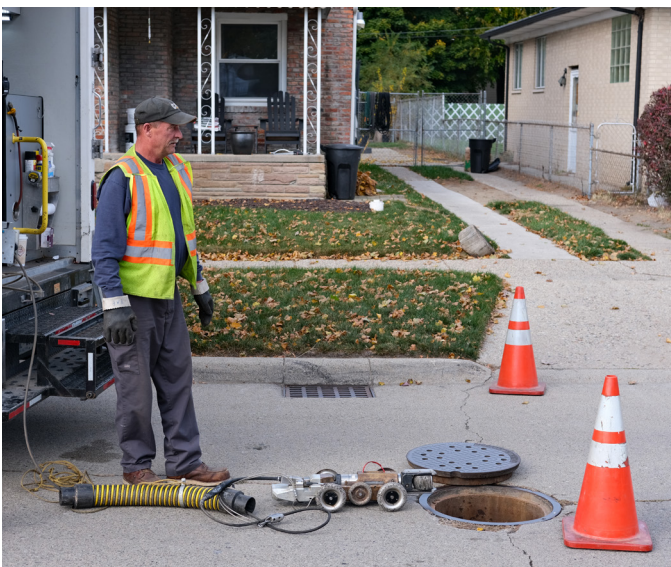
Maintenance Mechanic II Tom Wittke uses a camera robot to inspect the condition of pipes in the Charter Township of Royal Oak.
