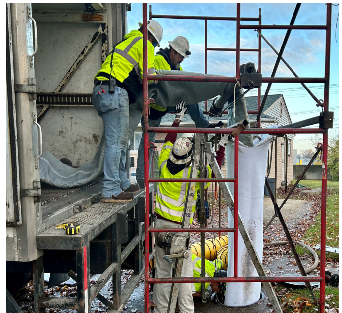
Crews inserting Cured-In-Place-Pipe lining into host pipe.
