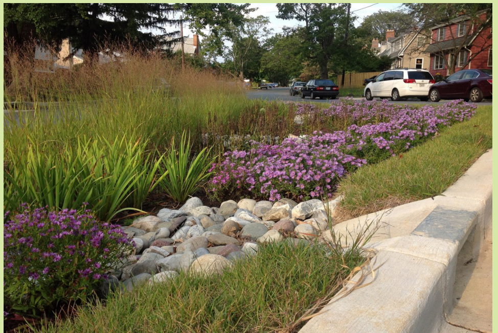
Pictured above: Rain garden and bioretention cell example.
