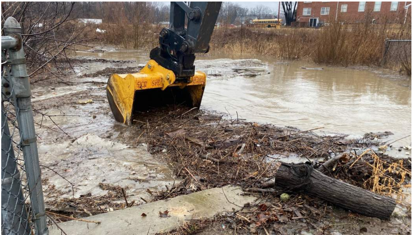
Debris and ice removal at inlet (looking west)
