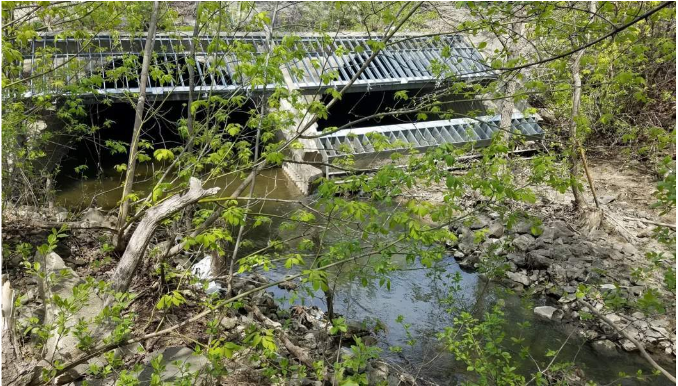
Outlet on South side of Big Beaver Road—Dual 12-x-8 feet Culverts
