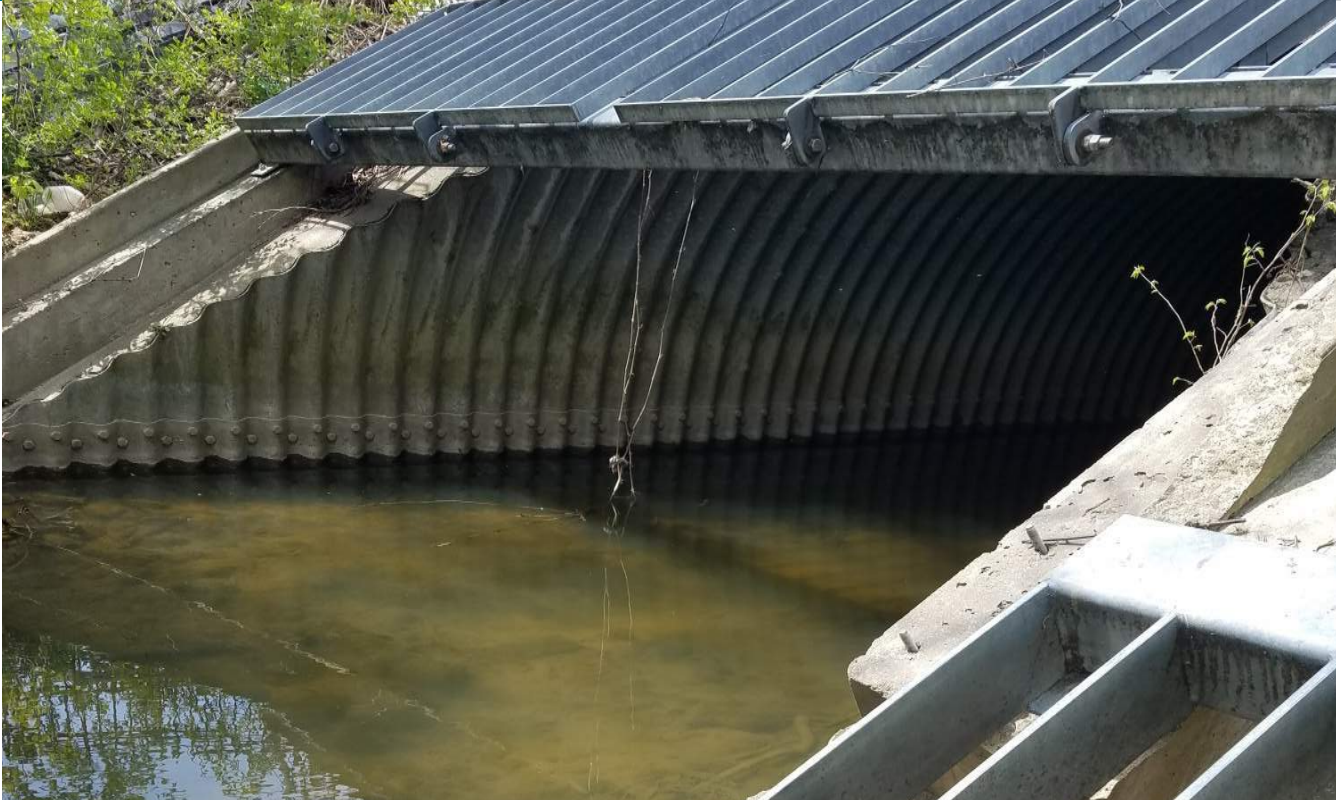
West Outlet Culvert Under Big Beaver Road—Less Debris
