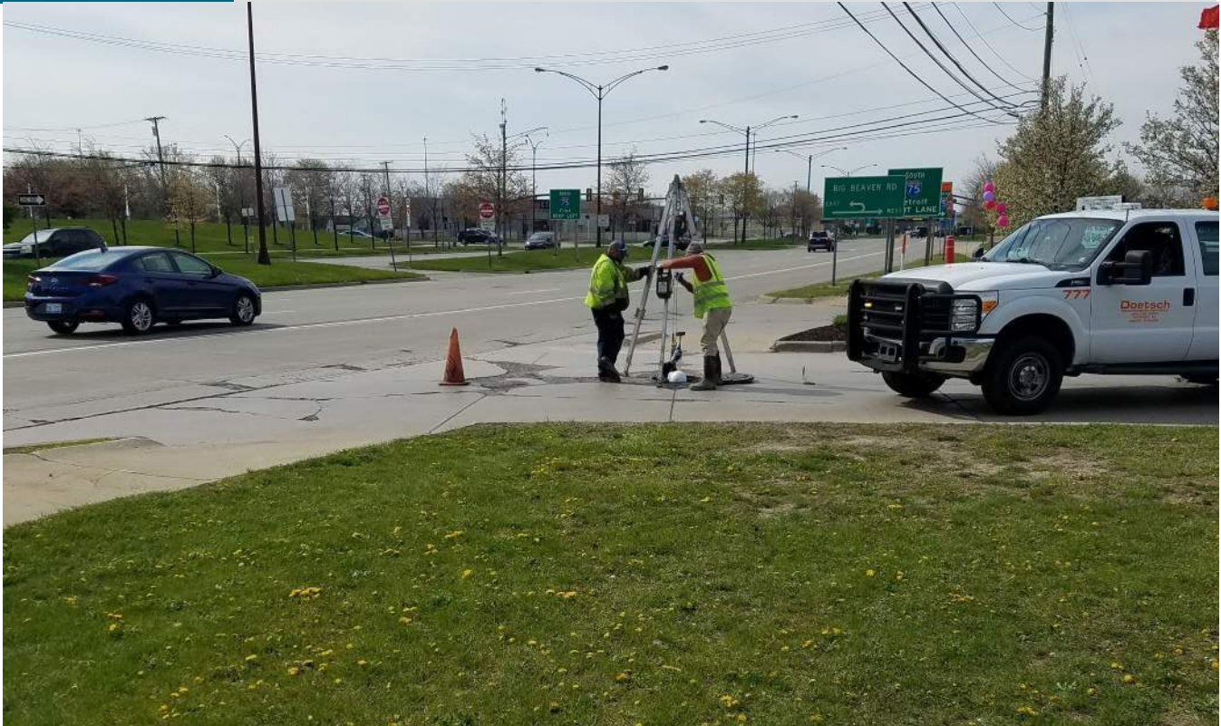
Stormwater Manhole Entry on West Rochester—Access Shaft into Rochester Road Culvert
