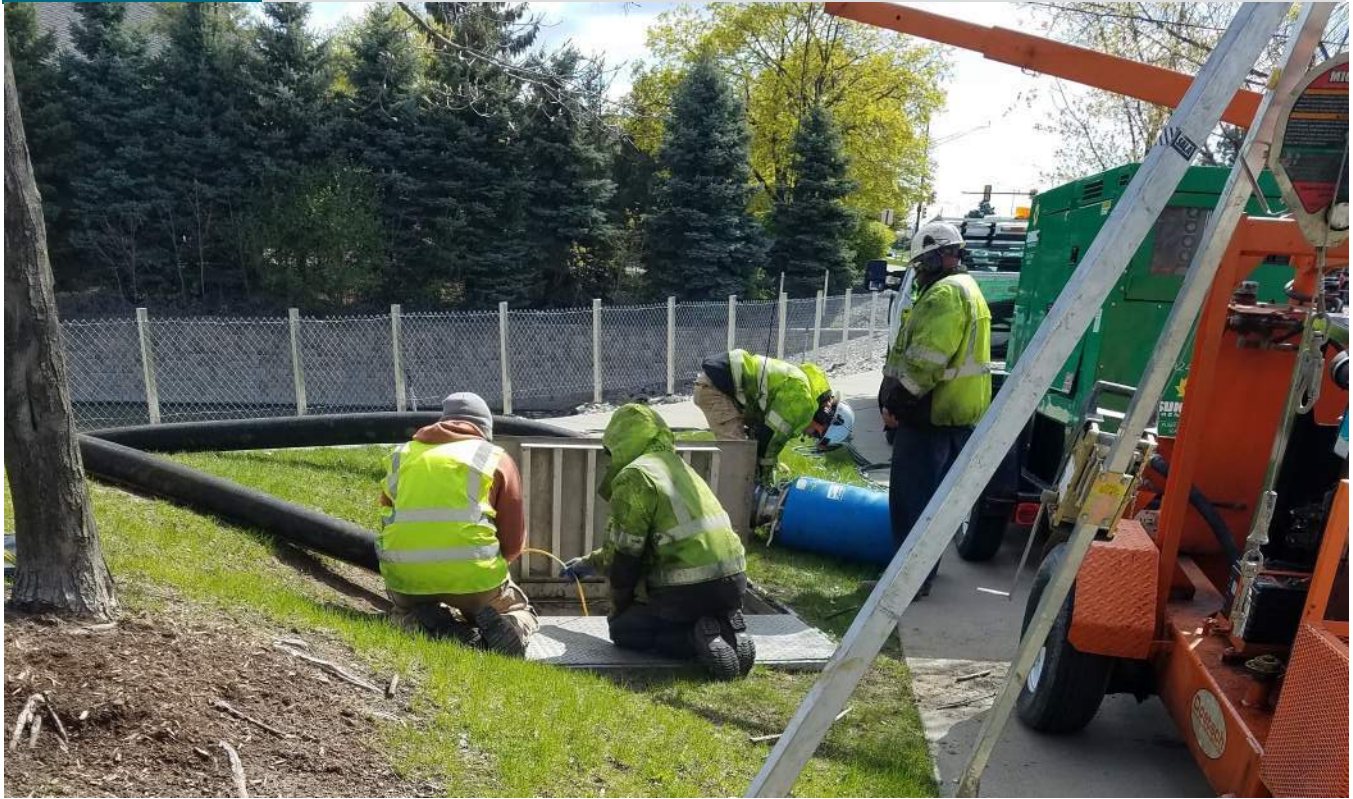
Lowering 6-inch Discharge Pipe Segments into Vault
