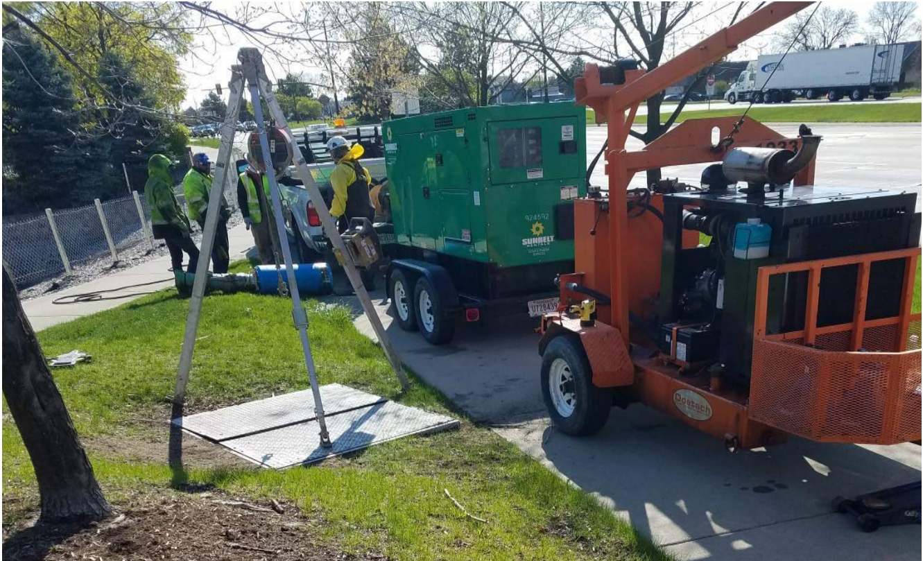
Preparing to lower 6-inch pump into vault
