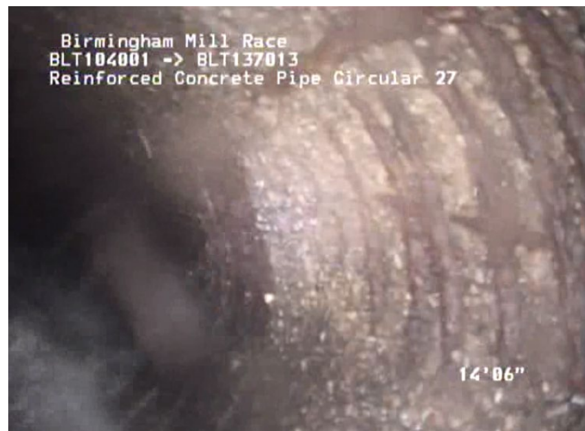
Exposed Reinforcement
