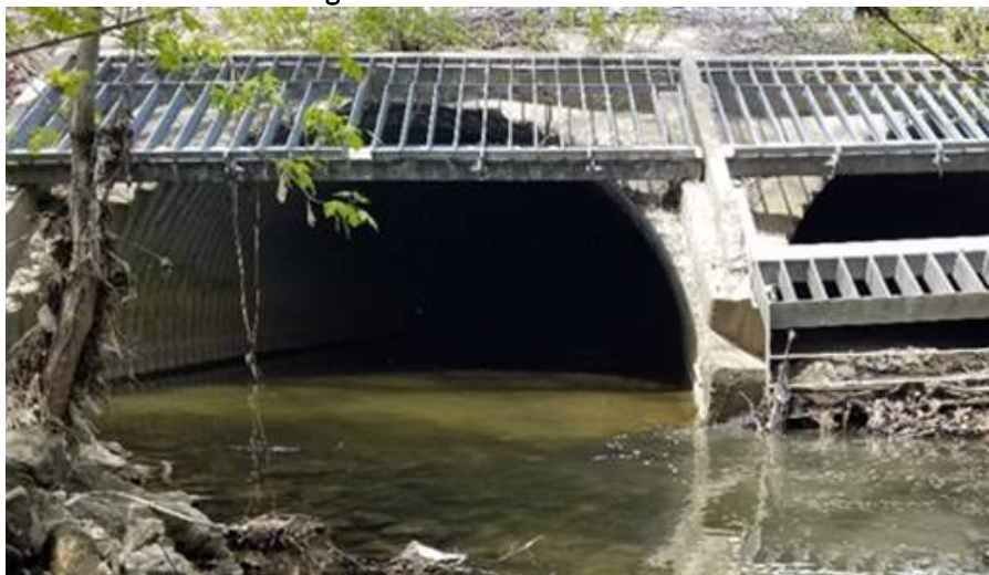
Figure 5 – Culvert Outlet Gate
