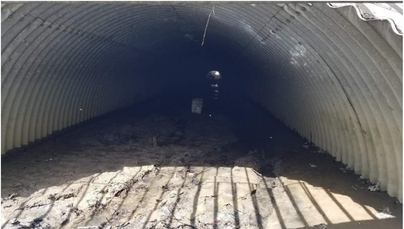
East Outlet Culvert with Layer of Debris on Bottom
