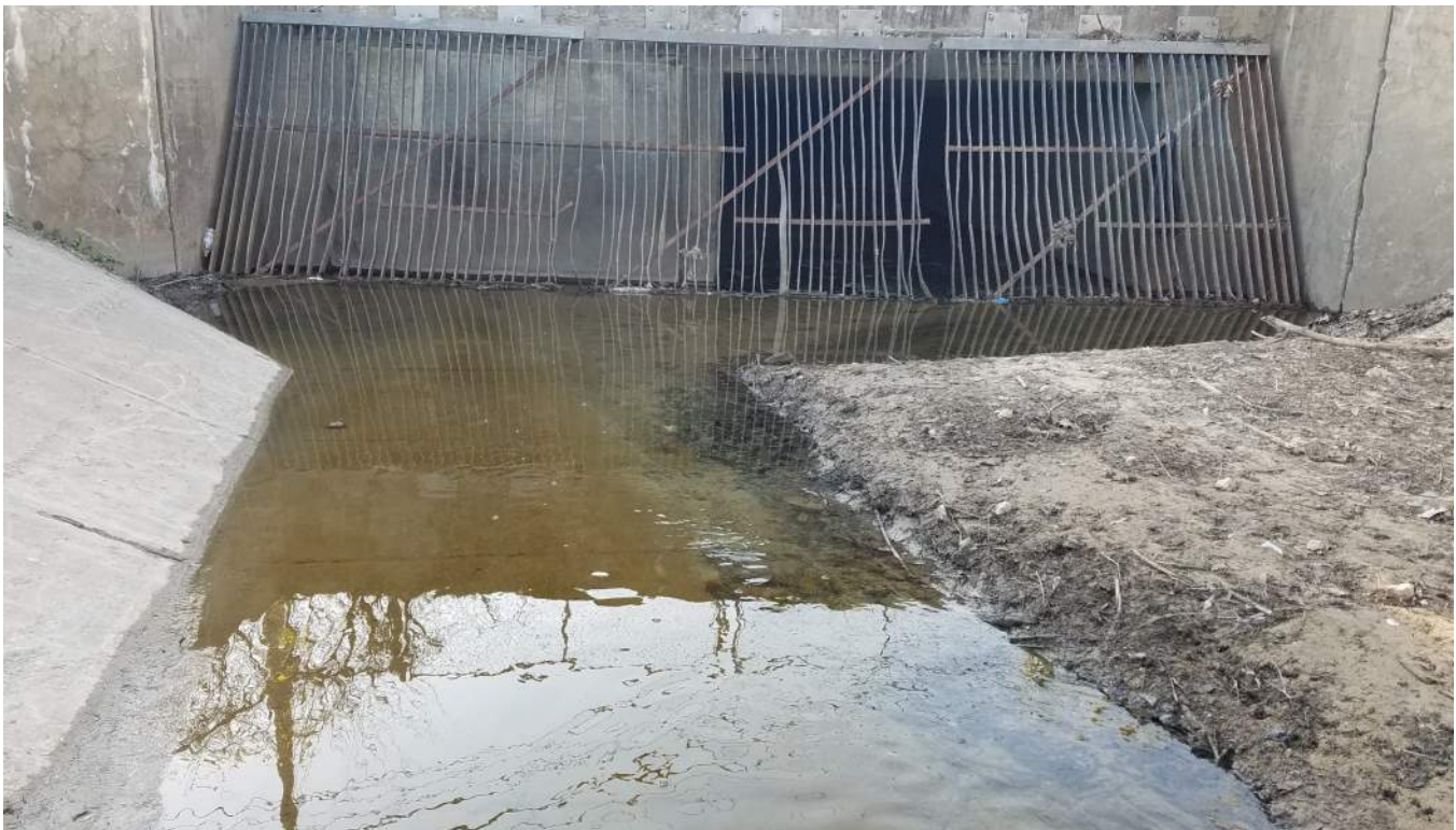
Sturgis Drain Inlet—Bulkheaded Left Side, Open Culvert on Right Side
