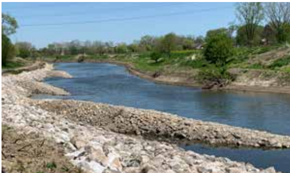
During strong or higher flow, especially after heavy rain, the three completed “J-hooks” at the Red Run Drain work in unison to prevent erosion of the drain bank by directing the flow toward the center of the channel.
