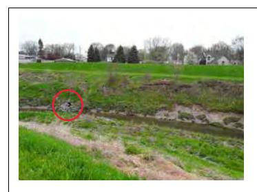
Inspect ID: 2022-0012 Title: 2704000028\_CELRE\_2022\_A\_0012\_2\_20220506T142447.jpg Rated Item: 4. Erosion Caption: Minimally Acceptable - Toe erosion. Outlet location noticed.
