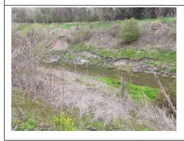
Inspect ID: 2022-0302 Title: 2704000028\_CELRE\_2022\_A\_0302\_1\_20220506T133909.jpg Rated Item: 4. Erosion Caption: Minimally Acceptable - Slope failures.
