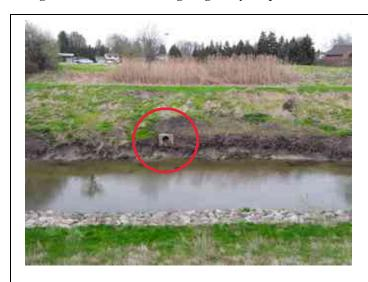
Inspect ID: 2022-0313 Title: 2704000028\_CELRE\_2022\_A\_0311\_1\_20220506T140545.jpg Rated Item: 4. Erosion Caption: Minimally Acceptable - Toe erosion. Outlet location also noted.
