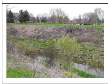
Inspect ID: 2022-0301 Title: 2704000028\_CELRE\_2022\_A\_0301\_1\_20220506T133537.jpg Rated Item: 4. Erosion Caption: Minimally Acceptable - Erosion, slope stability. Overly steep slopes with past failures.
