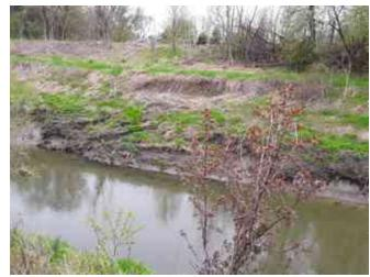
Inspect ID: 2022-0315 Title: 2704000028\_CELRE\_2022\_A\_0315\_1\_20220506T140928.jpg Rated Item: 4. Erosion Caption: Minimally Acceptable -Bank failure.
