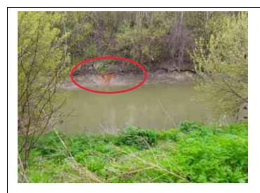
Inspect ID: 2022-0332 Title: 2704000028\_CELRE\_2022\_A\_0332\_1\_20220506T153345.jpg Rated Item: 4. Erosion Caption: Minimally Acceptable - Toe erosion and rust colored seepage noted.
