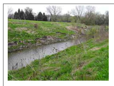
Inspect ID: 2022-0306 Title: 2704000028\_CELRE\_2022\_A\_0306\_1\_20220506T135225.jpg Rated Item: 4. Erosion Caption: Minimally Acceptable - Toe and bank erosion.
