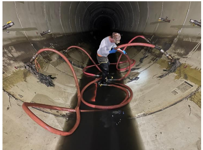
Channeline grouting in progress
