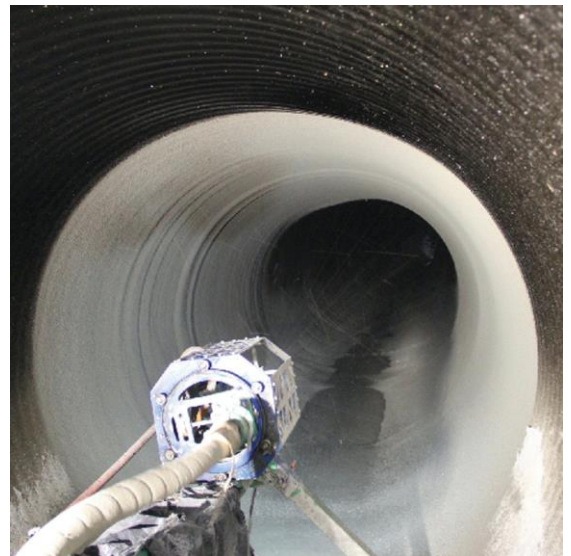
Figure 8: Spray application of a geopolymer lining
