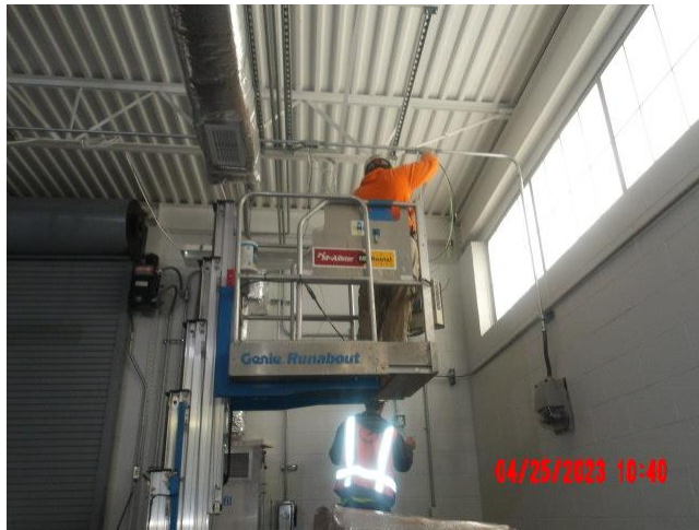
Contractor installing new ceiling lights in new electrical building area
