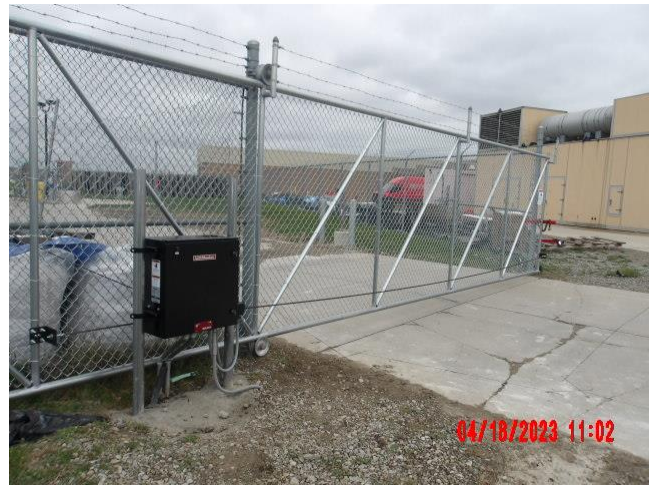
New sliding gate and gate operator
