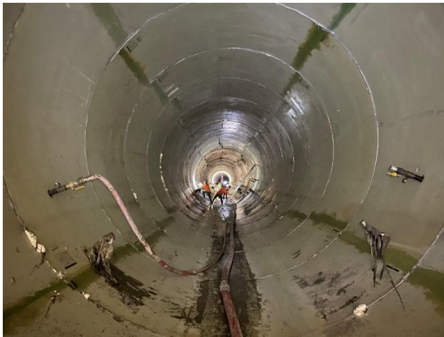
Channeline grouting in progress
