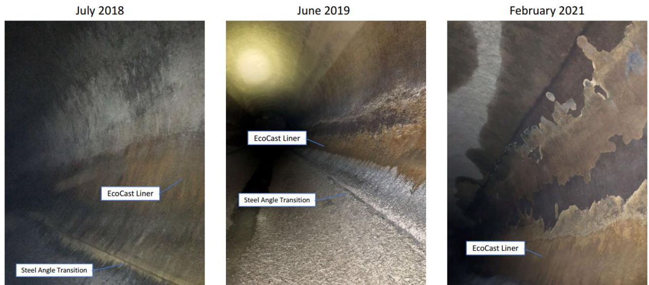
Figure 3: Stills from PCI-4 inspections (previously rehabilitated section)
