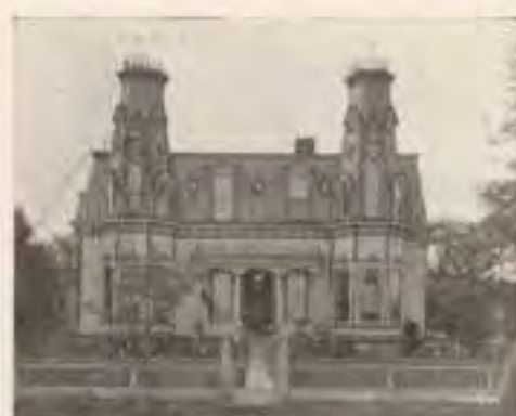
RESIDENCE OF JULIUS CARPENTER.
