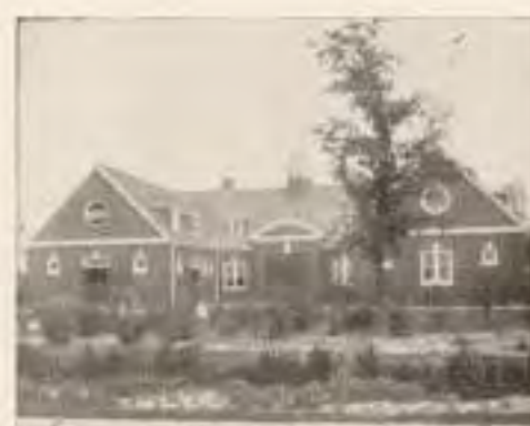
STABLES ON BRIARBANK FARM, W. T. BARBOUR, PROPRIETOR, BIRMINGHAM, MICH.
