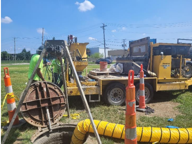
Spray-lining manhole MH-PCI-4-105
