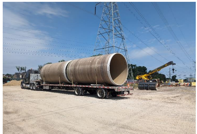
Delivery of Hobas pipe sections
