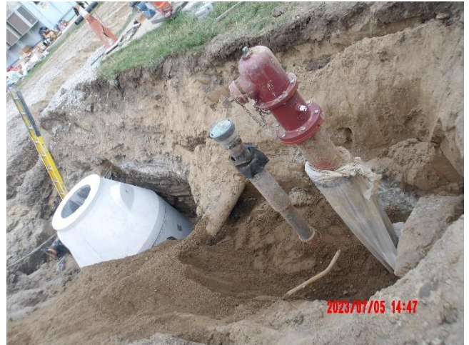
Relocation of fire hydrant
