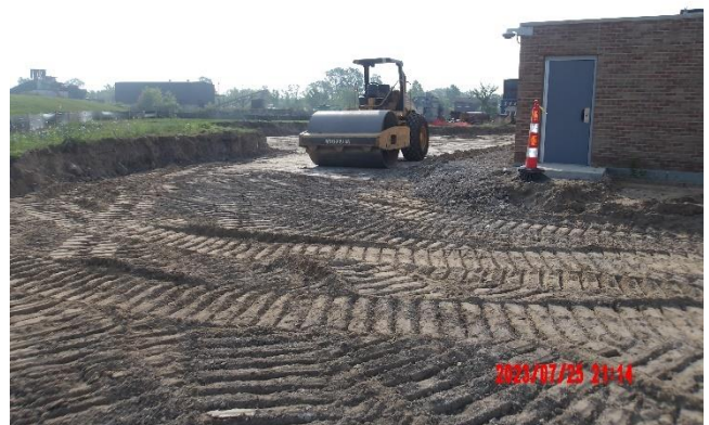
Excavating to subgrade for new concrete pavement
