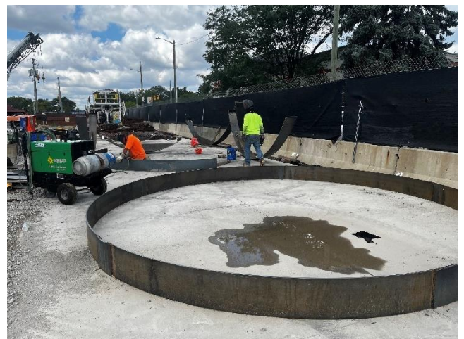
Welding RockHard pipe bracing
