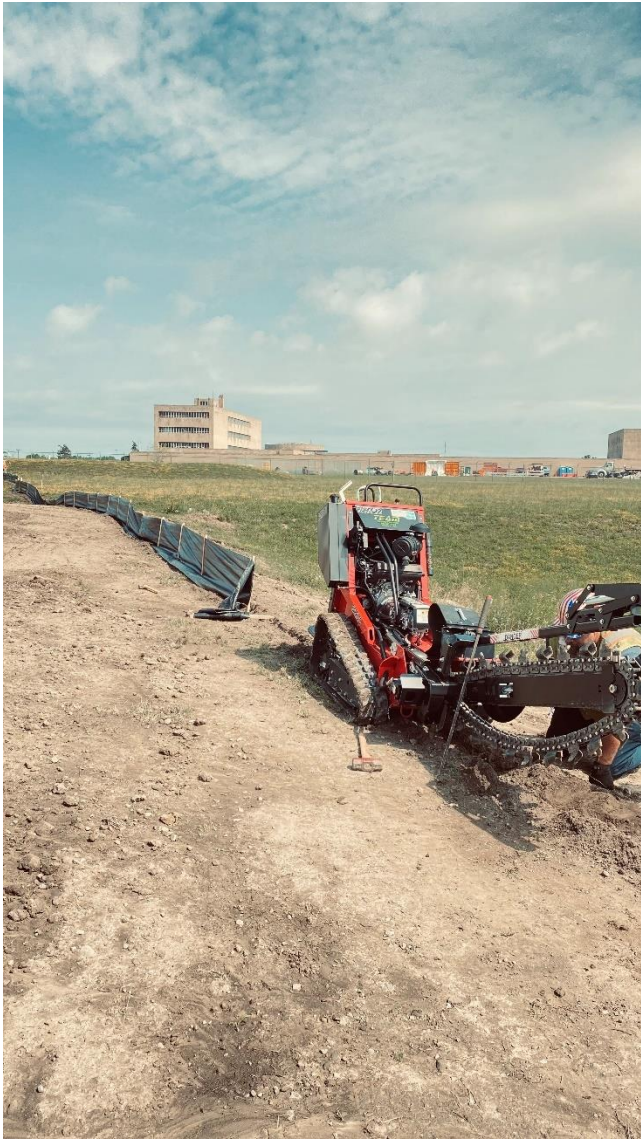
Silt fence installation
