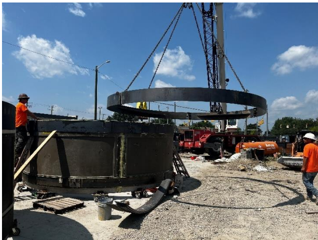
Installation of RockHard internal bracing
