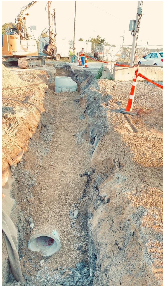
Installation of storm structures
