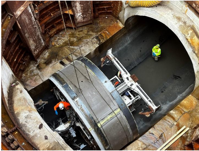
Lowering RockHard pipe section #1 for install
