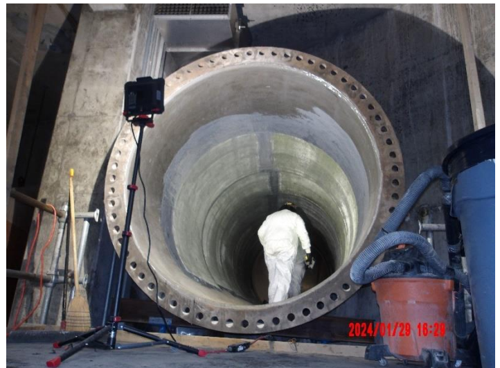
Contractor installing the second layer of Pump 5 Quake-wrap discharge pipe lining
