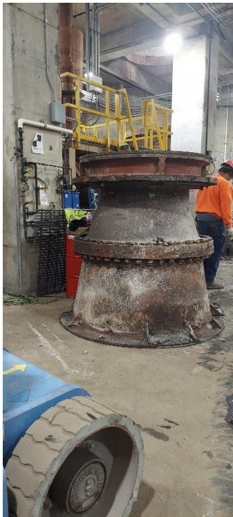
Removal of Sanitary Pump #5
