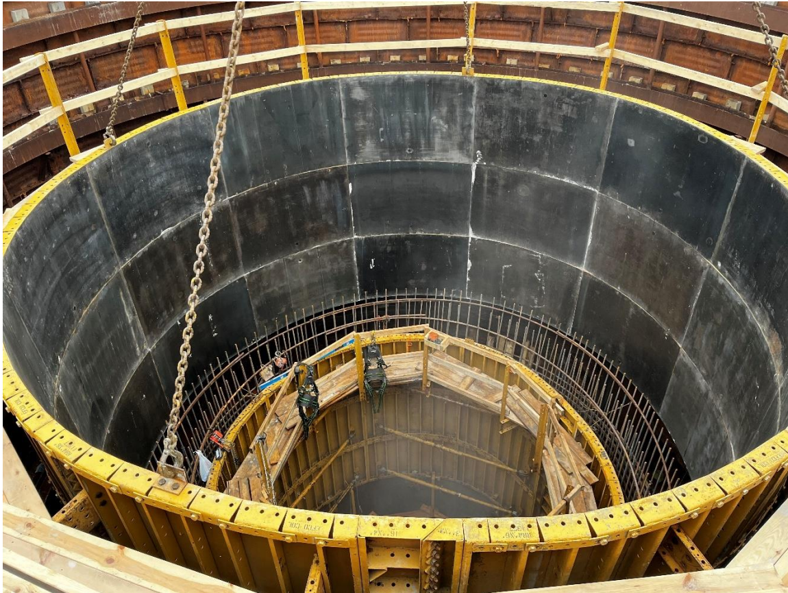
Installation of EFCO formwork prior to pouring
