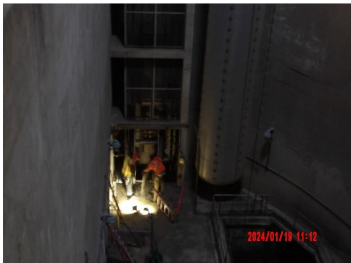
Contractor demolishing the existing wet well elevator frame
