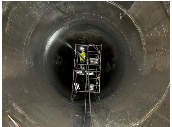
Application of shotcrete to RockHard transition section
