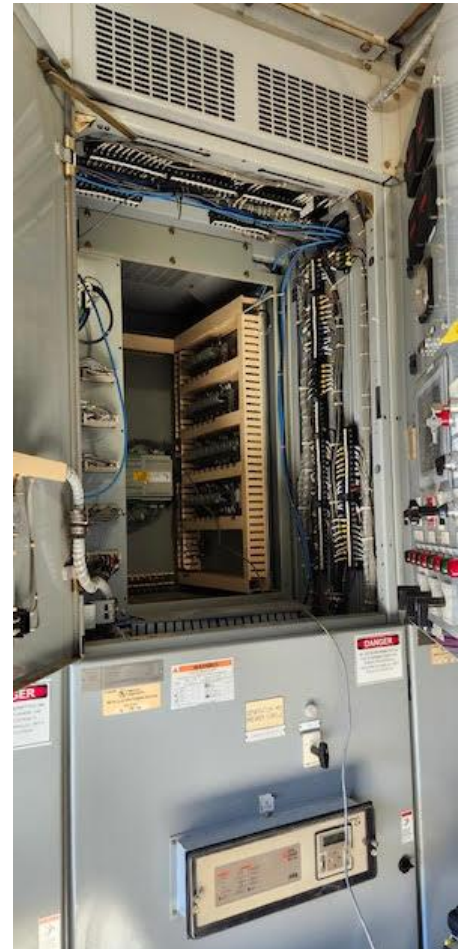
Finishing DSLC-2/MSLC-2 Upgrade
