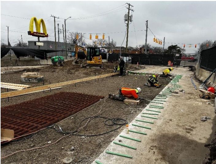
Preparing for pavement replacement
