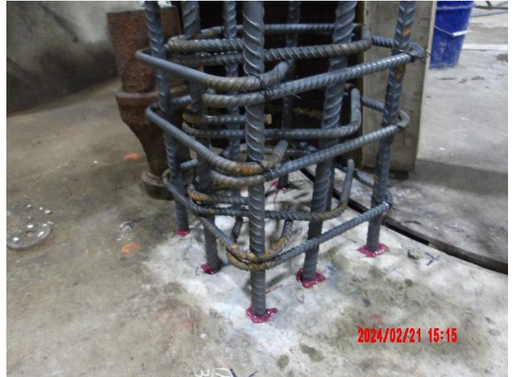
Assembly of Pump #5 pedestal reinforcement
