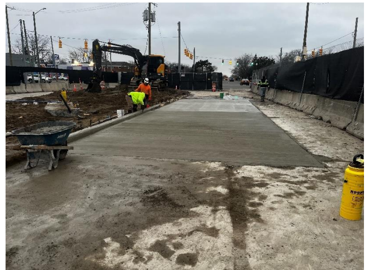
Finishing pavement replacement
