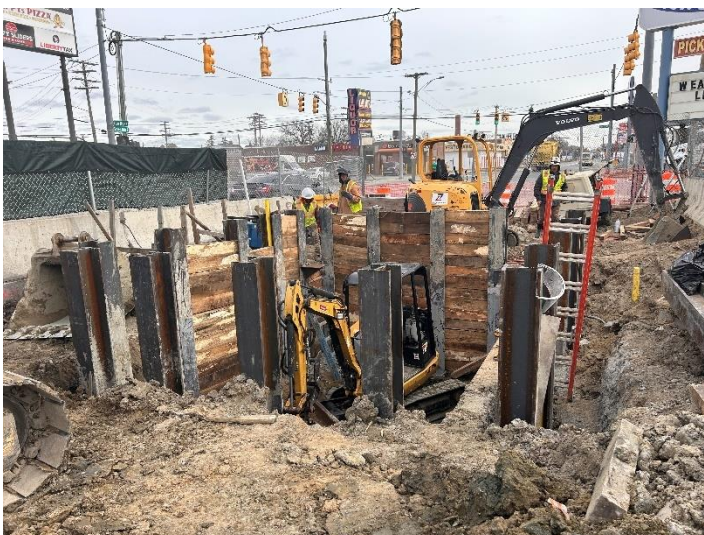
Progress on Temporary Earth Retention System
