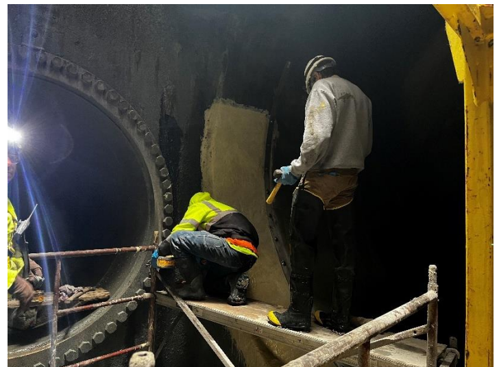
Armoring the transition of the discharge chamber
