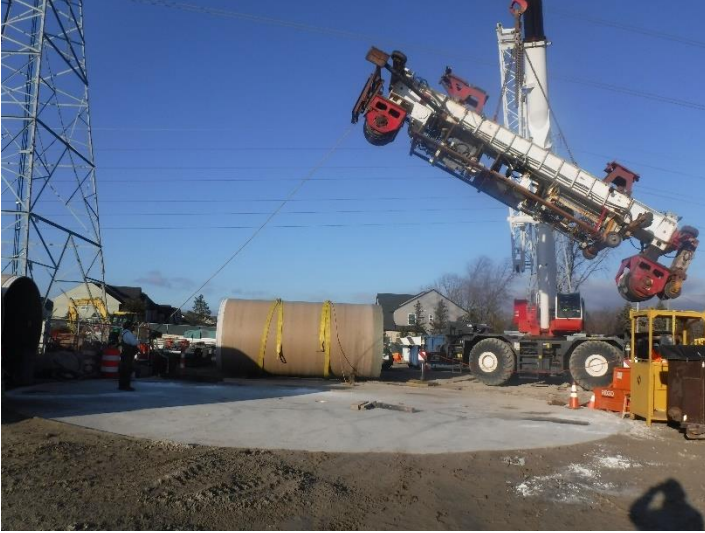
Positioning pipe carrier for lining operations
