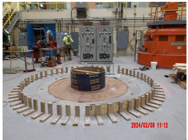
Construction of Pump #5 concrete footing
