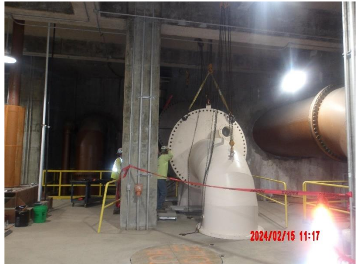
Installing 90° elbow at Pump #5
