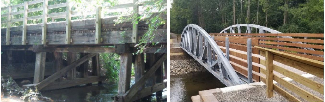
Photos: Existing bridge (left) to be replaced with single-span, 70' steel truss bridge similar to Paint Creek Trail Bridge 33.7 (right)
