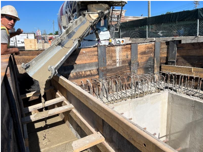
Placing flow fill at south side of access structure
