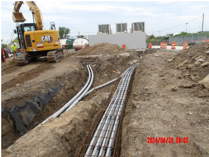
Installing duct bank for new conduit runs
