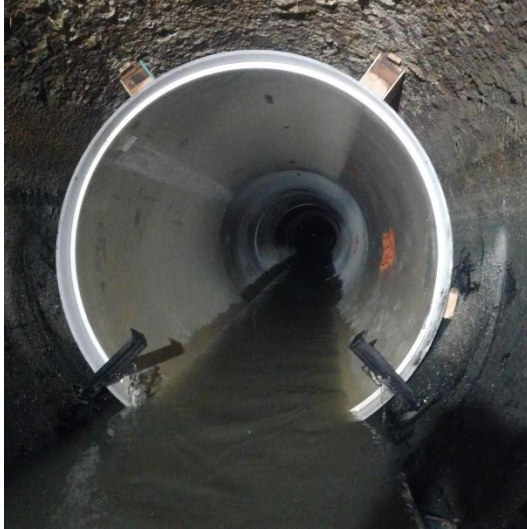
Installed Hobas liner
