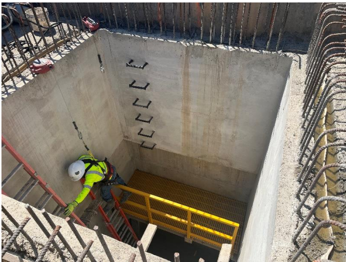
Installing FRP platform in 7 Mile access shaft structure
