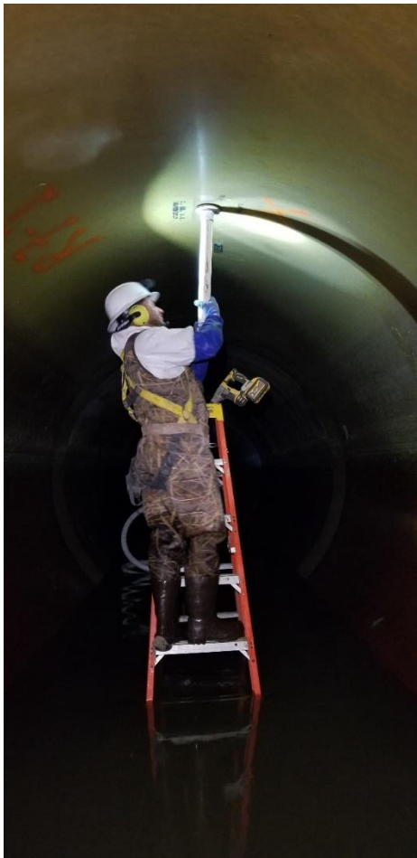
Annulus grouting operations
