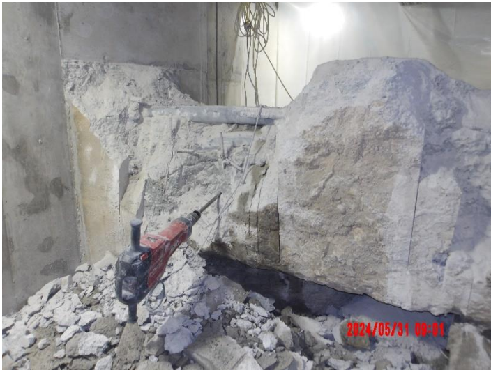
Demolition of existing electrical case in basement of new electrical building
