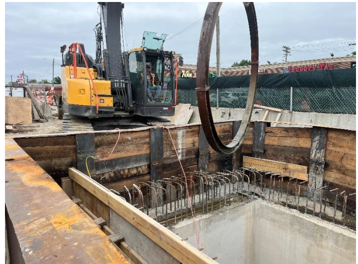
Removing temporary support ribs from 8 foot adit sewer
