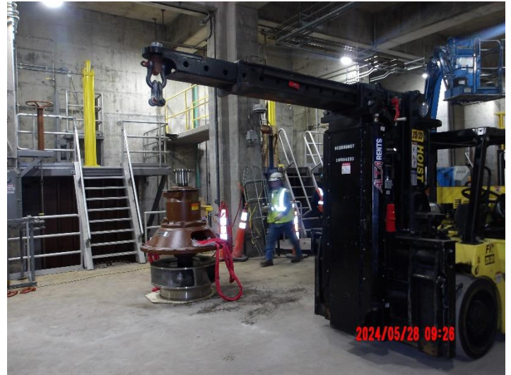
Swapping interior moving parts between Pumps #5 and 6
