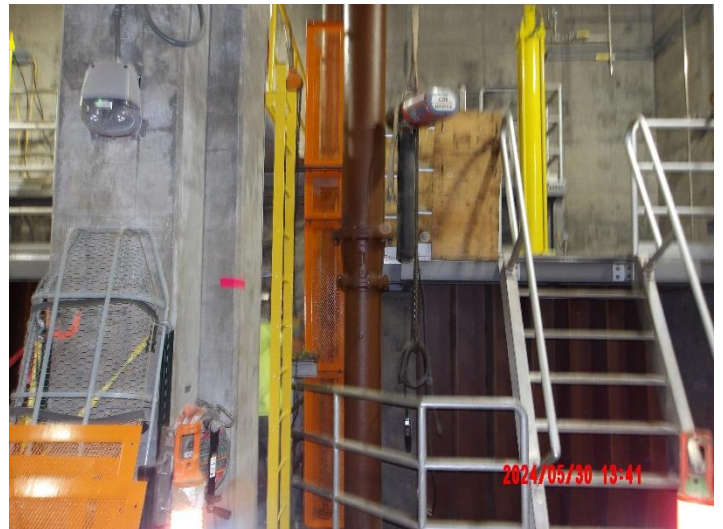
Installation of draining pump drive shaft on 6 th floor
