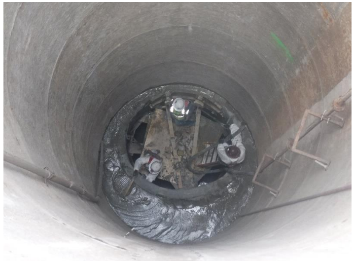
Construction of MH-5 riser
