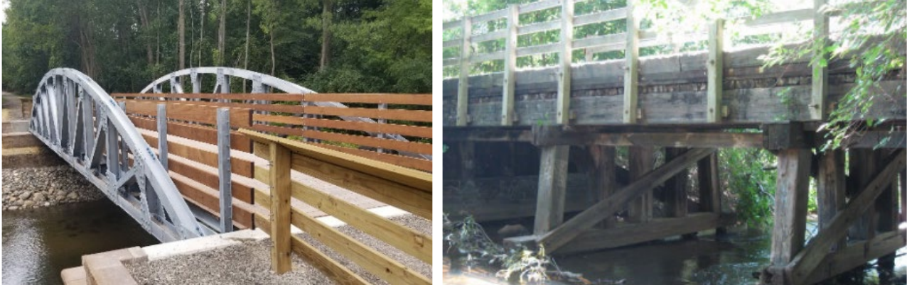
Photos: Existing bridge (left) to be replaced with single-span, 70' steel truss bridge like Paint Creek Trail Bridge 33.7 (right)
