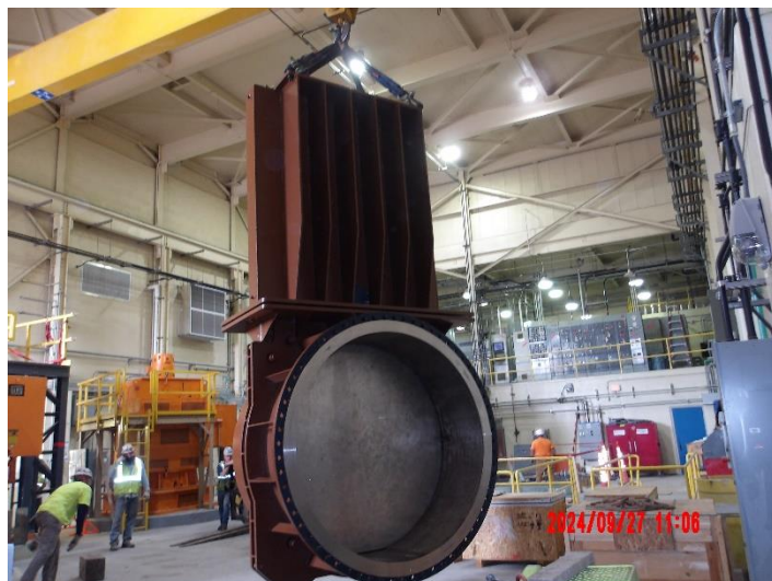
Staging new Knife Gate Valve 6 on 6 th floor
