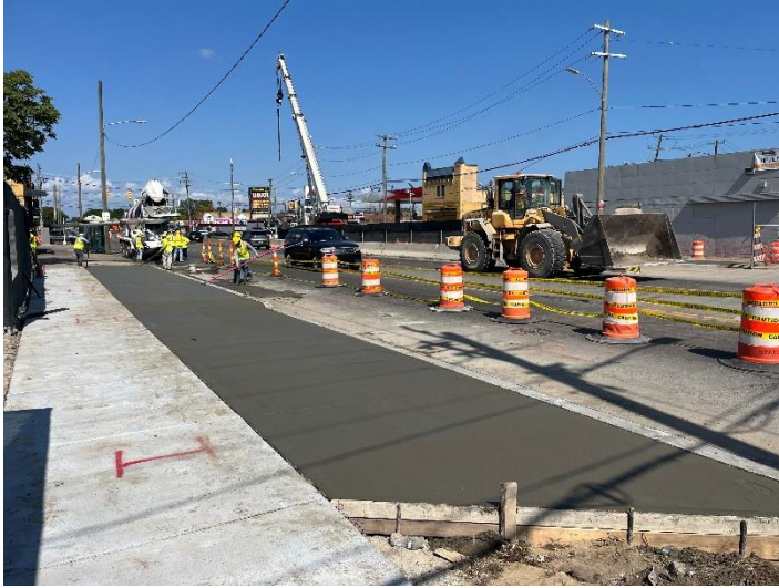
Finishing sidewalk concrete, southbound Van Dyke Road
