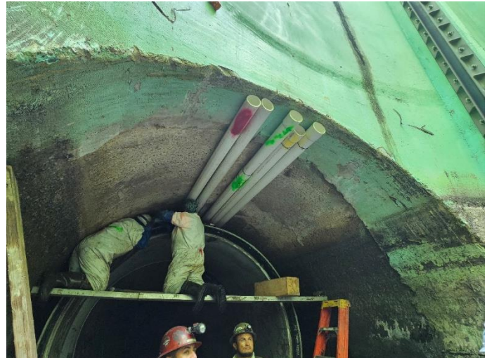
PVC pipes at crown at CS-12 shaft for placing annular grout
