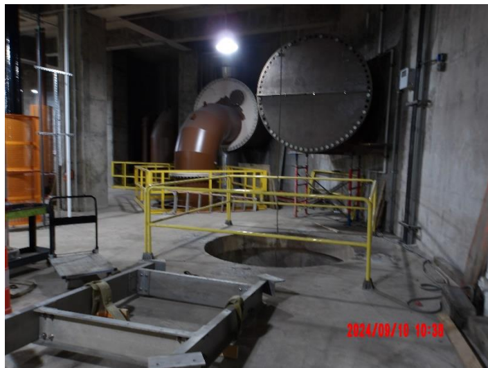
Vertical pipe restraint assembly for Pump #6 discharge
