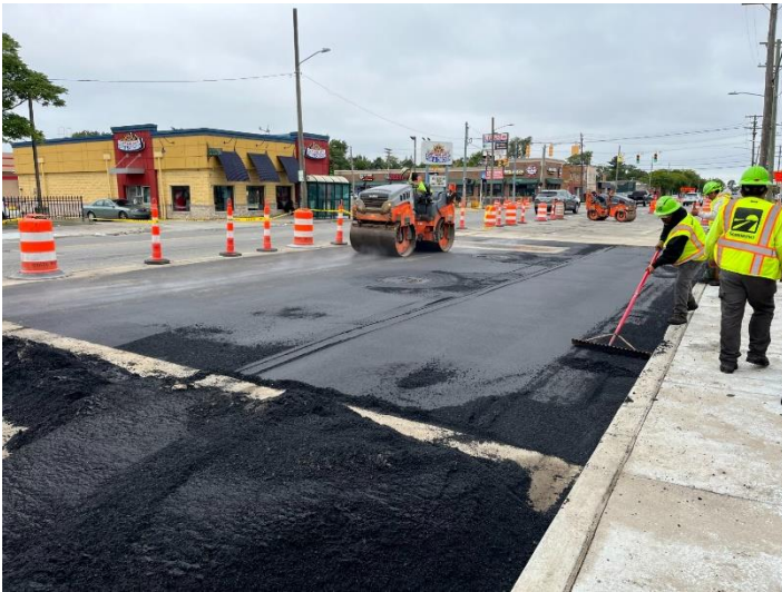
Van Dyke Road asphalt placement
