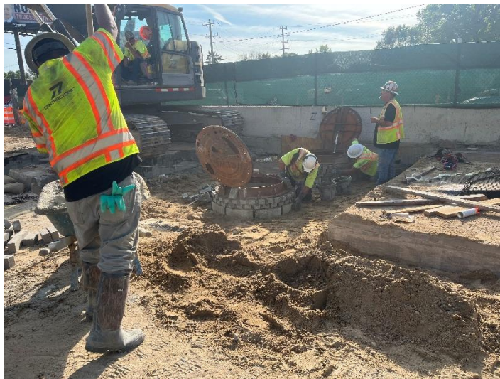
Contractor placing new manhole risers and covers
