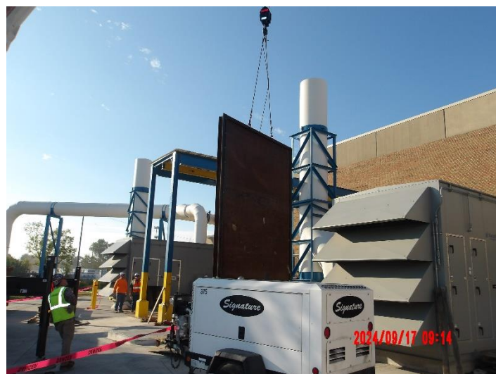
Lowering stop log at the north wet well in preparation for Knife Gate Valve 6 replacement
