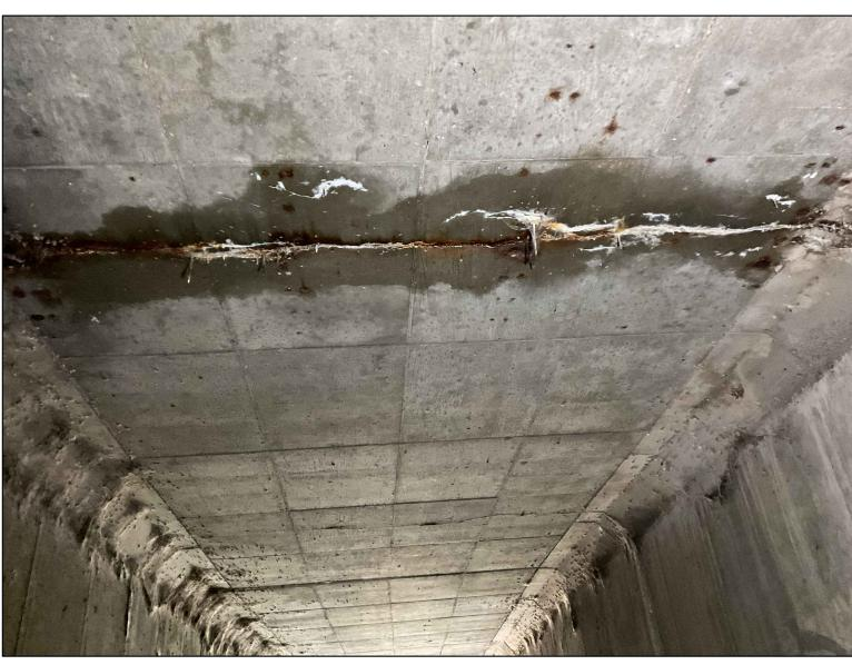
PHOTO 7: PRESSURE INJECTION OF WEEPING CRACKS REPAIR TYPE 2B - CULVERT TOP SLAB
