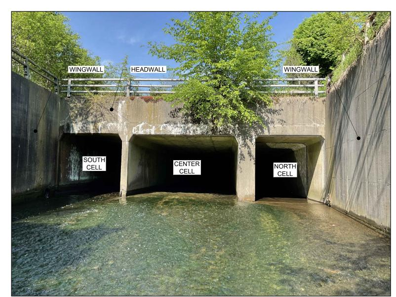
PHOTO 1: OUTLET STRUCTURE (LOOKING WEST)
