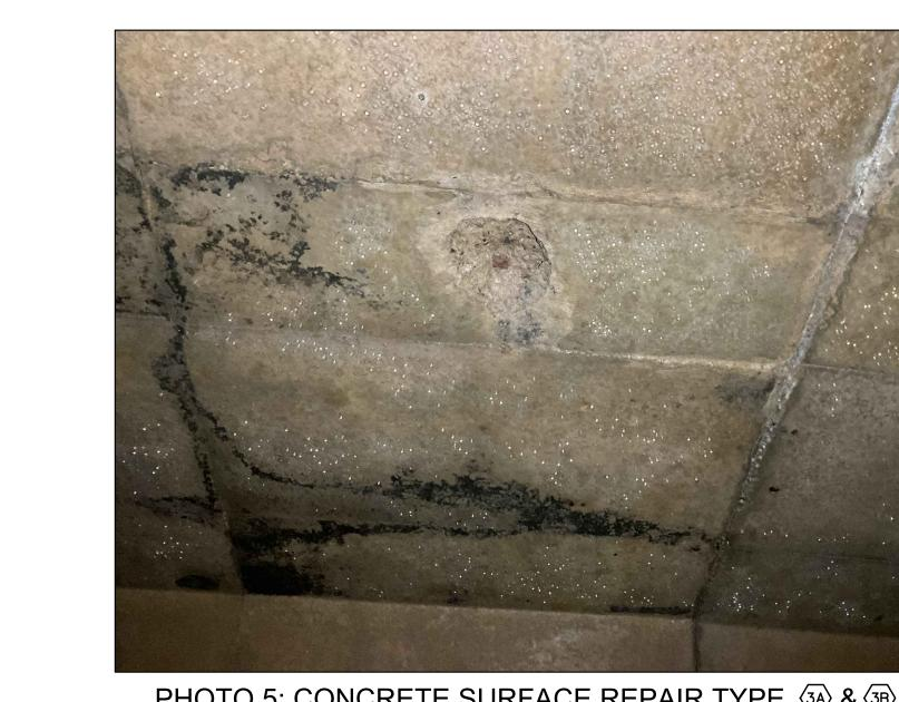
PHOTO 5: CONCRETE SURFACE REPAIR TYPE 3A & 3B -CULVERT TOP SLAB
