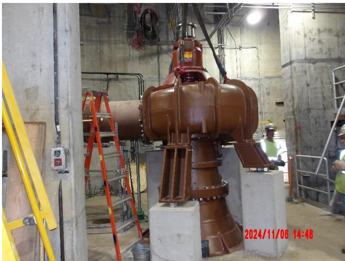
Installation of Pump #6
