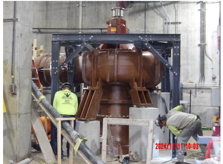
Installation of Pump #6
