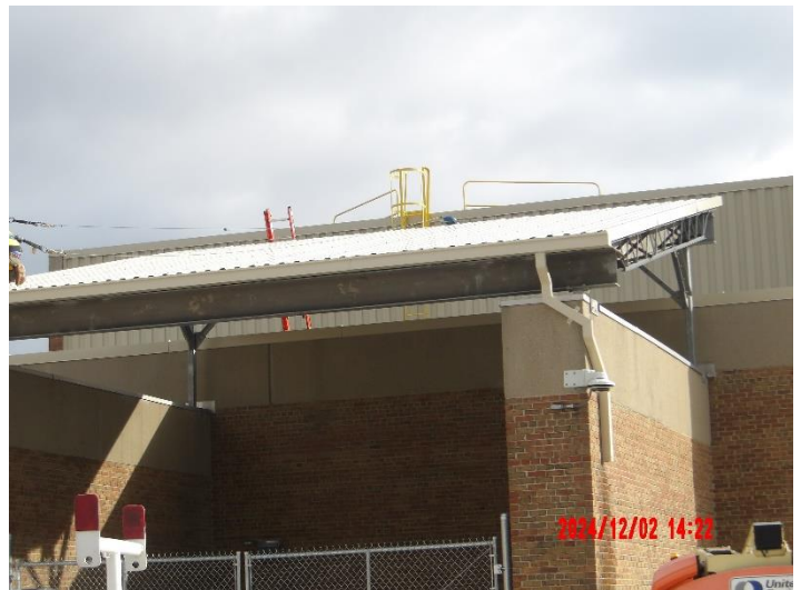
Gutter and downspouts of new metal roofing system
