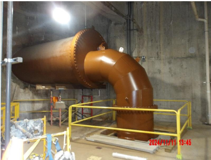
Freshly painted Pump #6 elbow on 3 rd floor
