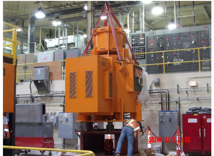
Installing Pump #6 electrical motor
