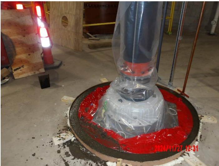
Pump #6 drive shafts after alignment with motor
