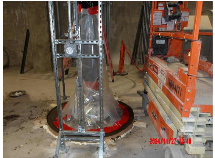
Pump #6 speed sensor and thrust bearing on 2 nd floor
