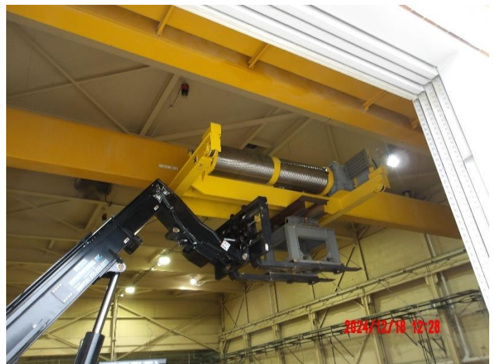
Removing existing trolley and hoist and installing new overhead crane elements
