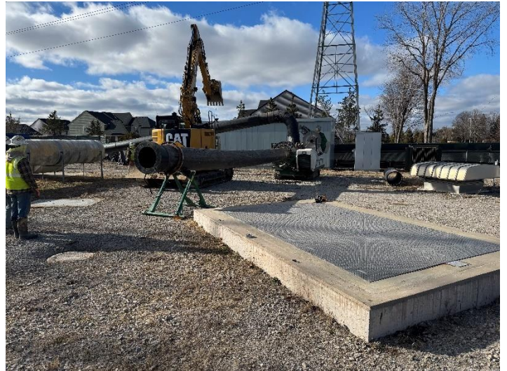
Contractor placing bypass equipment at CS-12
