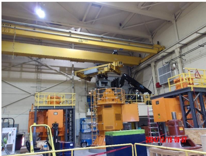
Removing existing trolley and hoist and installing new overhead crane elements
