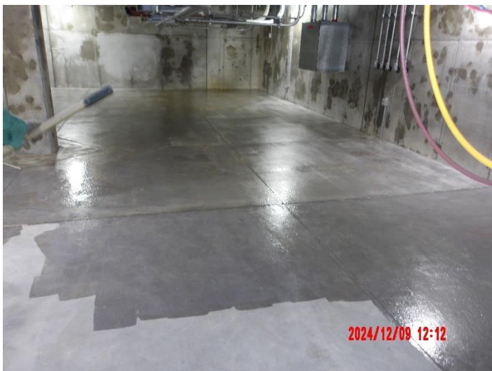
Seal coating the new electrical building
