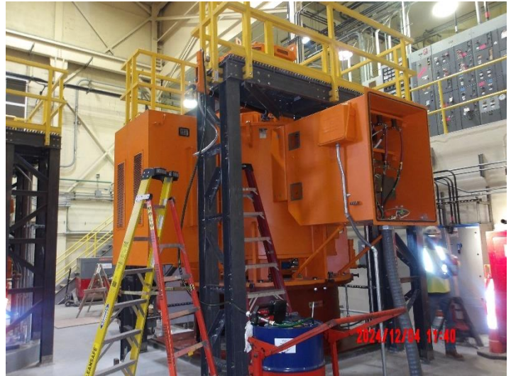
Installing Pump #6 top platform guard rails
