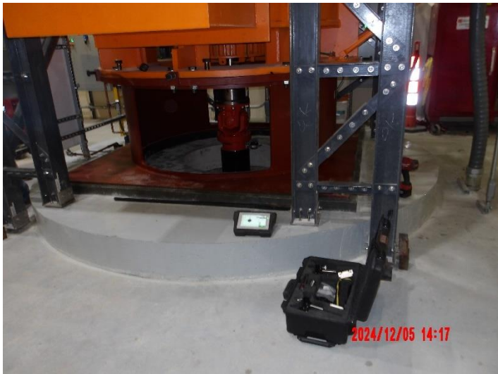
Final laser-alignment of Pump #6
