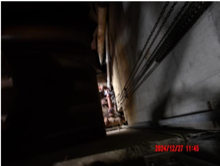
Installation of 4-inch for KGV draining system at Pump #6
