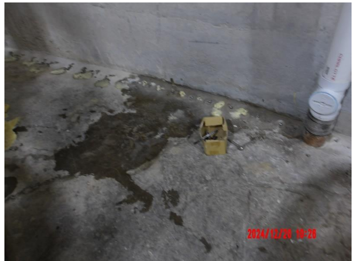
Sealing infiltration at caisson wall
