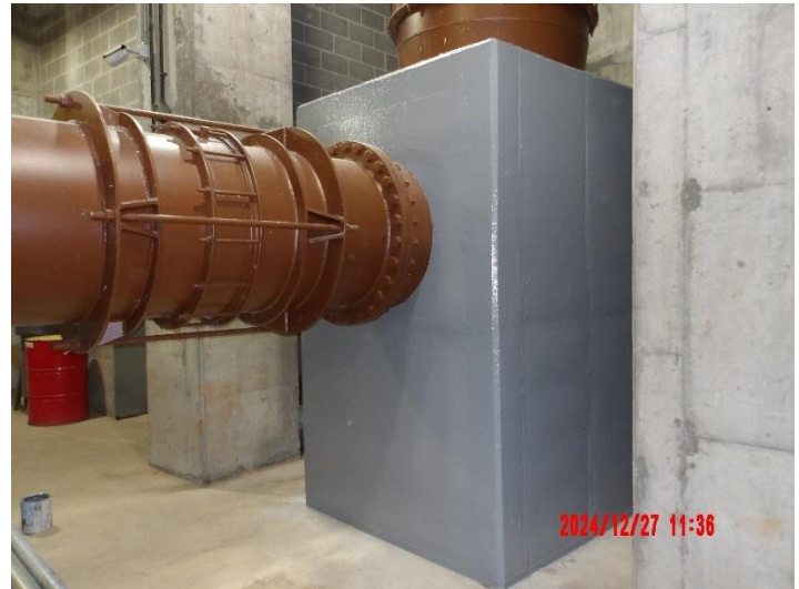
Fresh paint on concrete thrust block at motor floor
