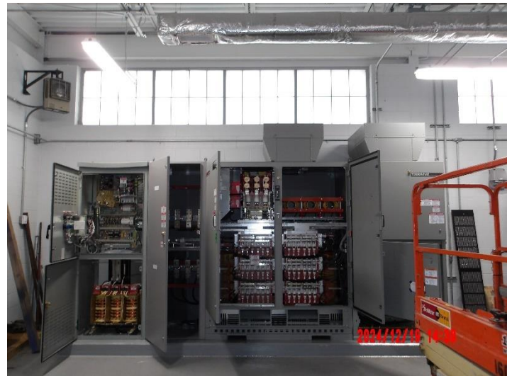
New Pump #4 VFD panel in electrical building
