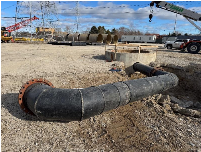
Contractor placing bypass equipment at CS-12
