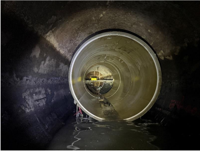
Slip lining in PCI-7
