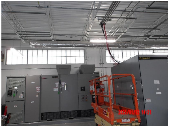
Installation of Pump #4 VFD in electrical building
