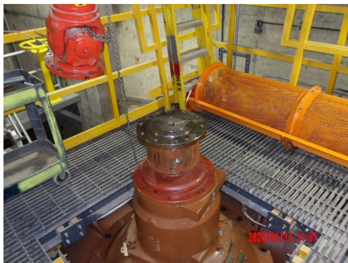
Swap of rotating assemblies at Pumps #1 & #3 repair leaks
