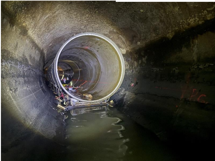
Slip lining in PCI-7
