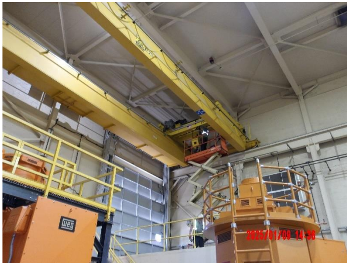
Completing installation of overhead crane
