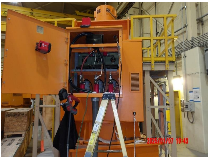
Connecting high voltage cable at Pump #4 excitor
