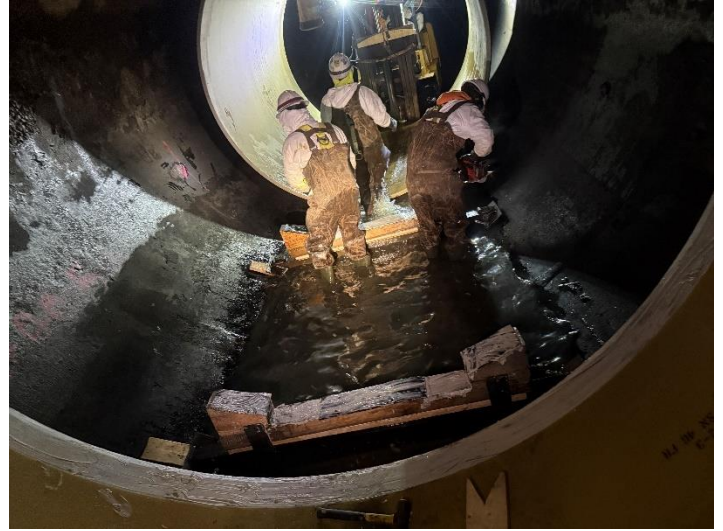
Slip lining in PCI-7
