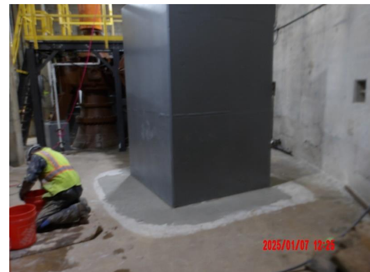
Prepping 6 th floor before final protective coat
