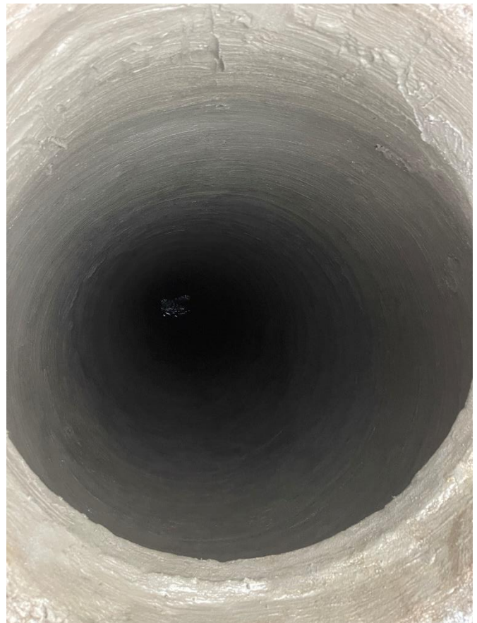
Spray lining of PCI-7-MH-111
