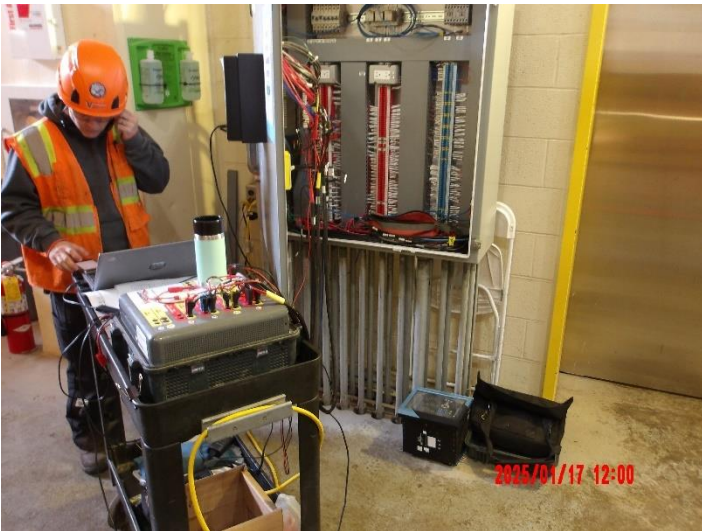
Inspecting Pump #4 wiring on first floor
