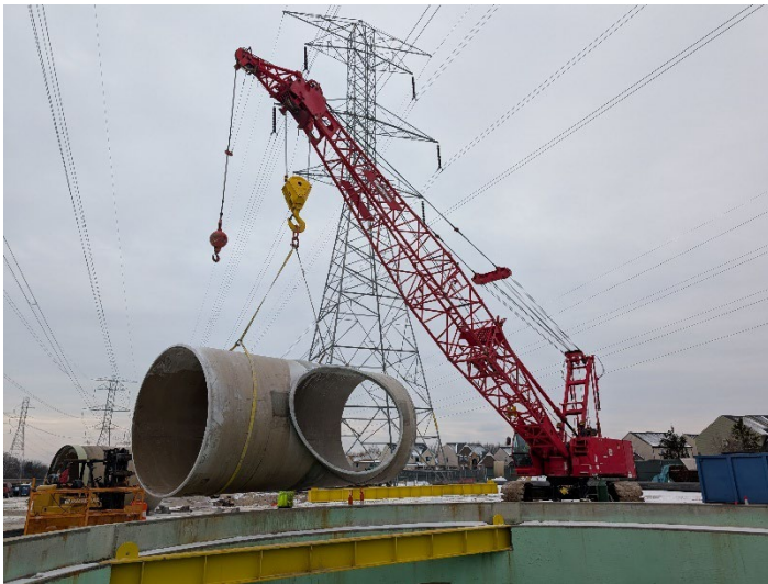
Lowering mitered slip-lining segment for PCI-7/8 connection
