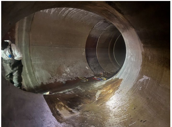
Mitered slip-lining section in-place at PCI-7/8 connection
