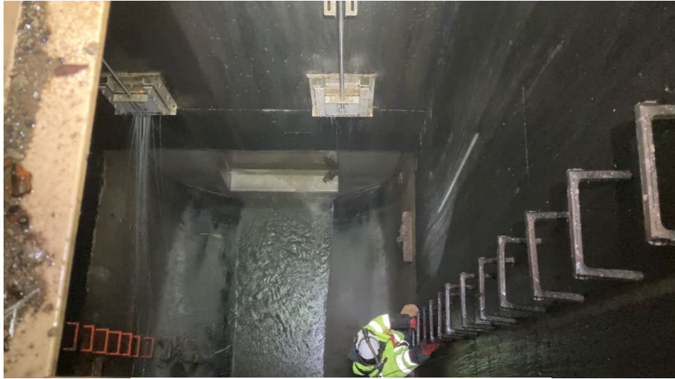
PC 663 bulkhead gate in operation
