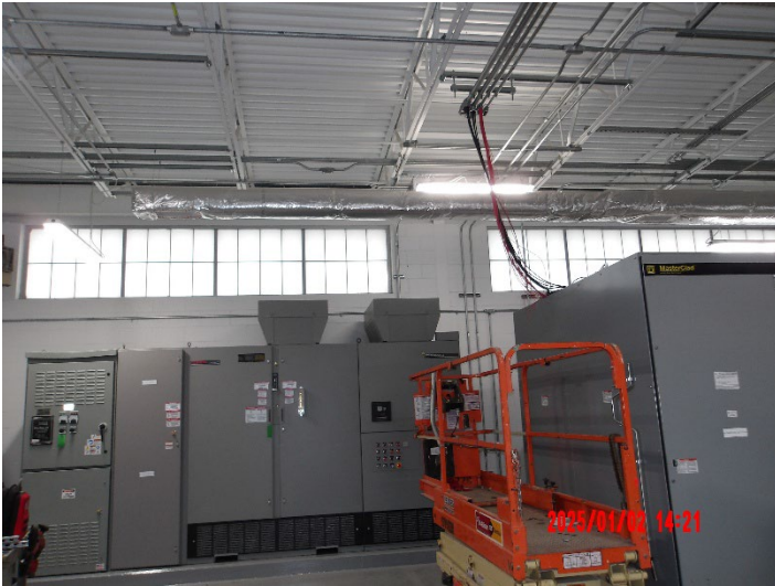
Installation of Pump #4 VFD in electrical building
