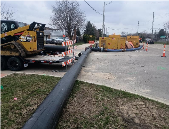
Bypass set-up at ST-S-3
