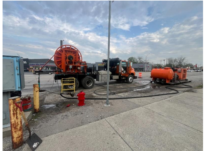
Topside PCI-19 jet-cleaning operations
