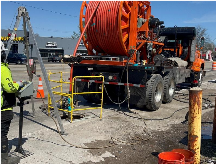
Topside PCI-19 jet-cleaning operations
