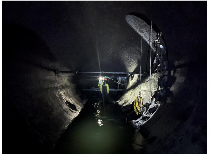
In-pipe preparation for sewer blocker for jet cleaning in PCI-19
