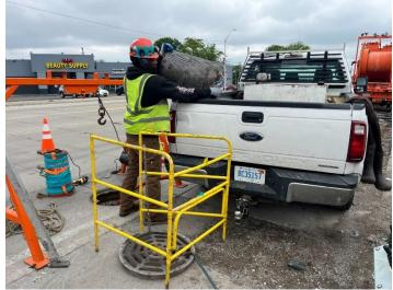
Manually removing debris via guard-rail winch
