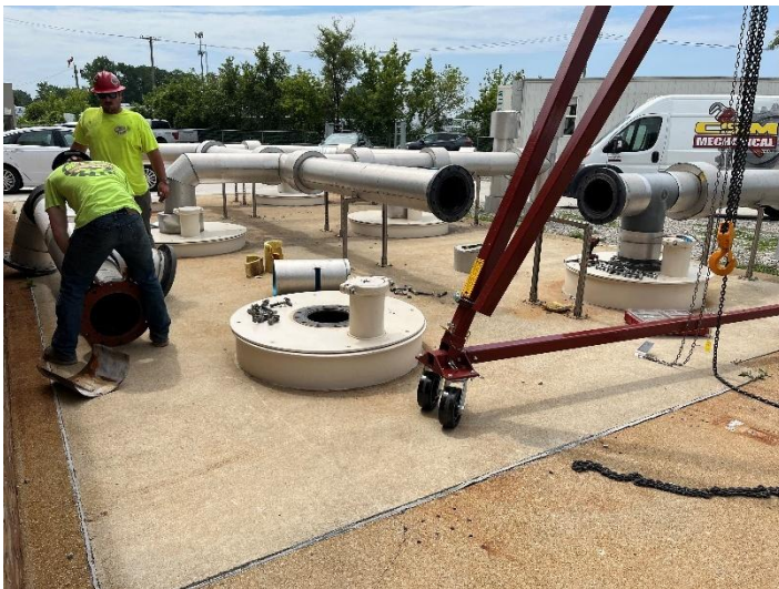
Dismantling of pipe insulation and Pump #4 piping
