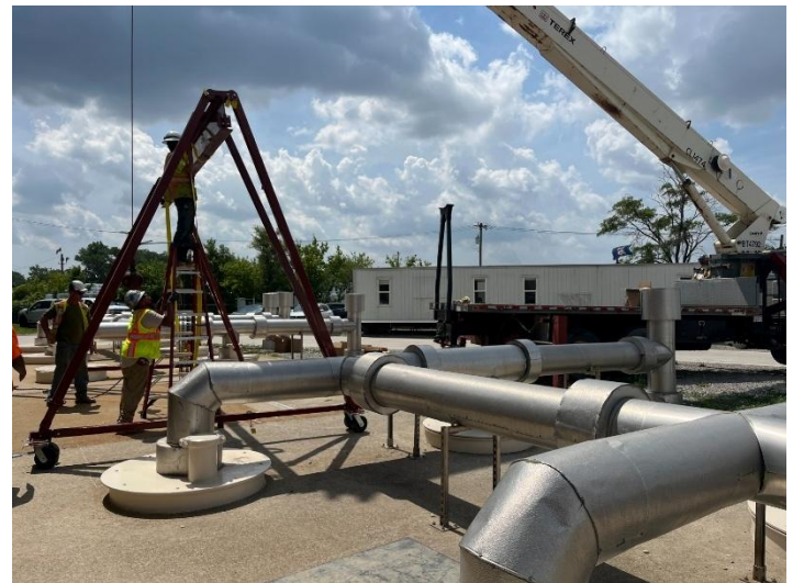
Installation of Wallace 5-ton gantry crane
