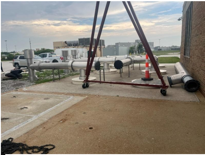
Blind flange installations at Pump #3
