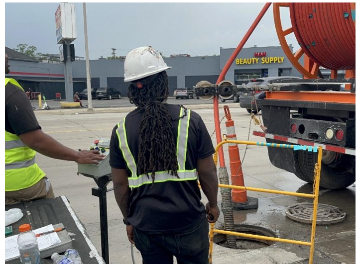
Topside set-up for jet cleaning
