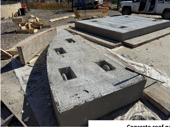
Concrete roof panels for CS-12 onsite
