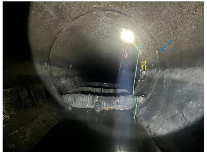
Grouted reach of PCI-19 and debris catcher (C2B)
