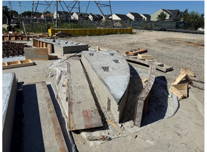
Concrete roof panels for CS-12 onsite
