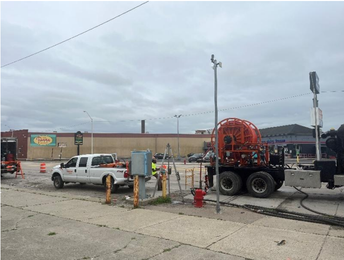
Topside set-up for jet cleaning at PCI-19-102 (C2B)
