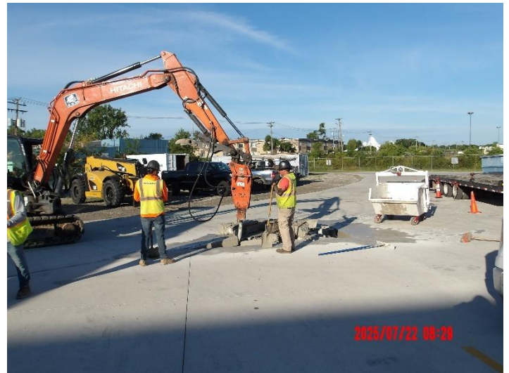
Repair of damaged concrete underway (NESPS Punchlist)
