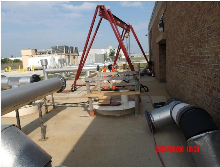
Installing backflow preventers in NESPS pump risers (related to NIEA C2B)
