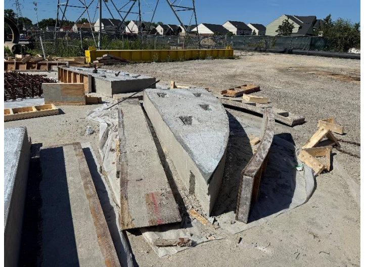
Concrete roof panels for CS-12 onsite
