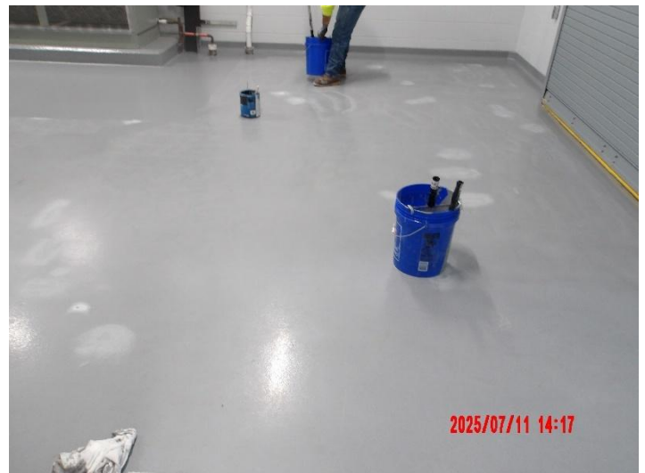
Epoxy coating repairs underway on floor of new electrical building (punchlist)
