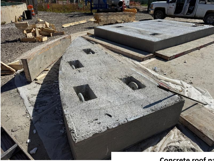
Concrete roof panels for CS-12 onsite
