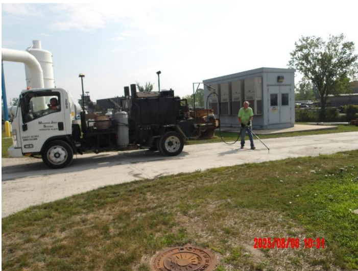
Placing rubber in joints of concrete drive (punchlist)
