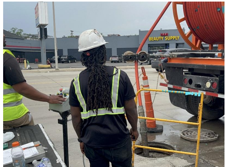
Topside set-up for jet cleaning
