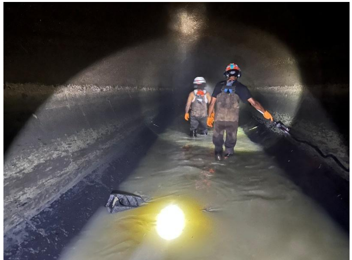
Inspection of cleaning progress at PCI-19
