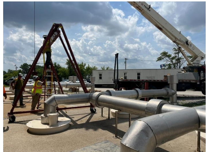
Installation of Wallace 5-ton gantry crane
