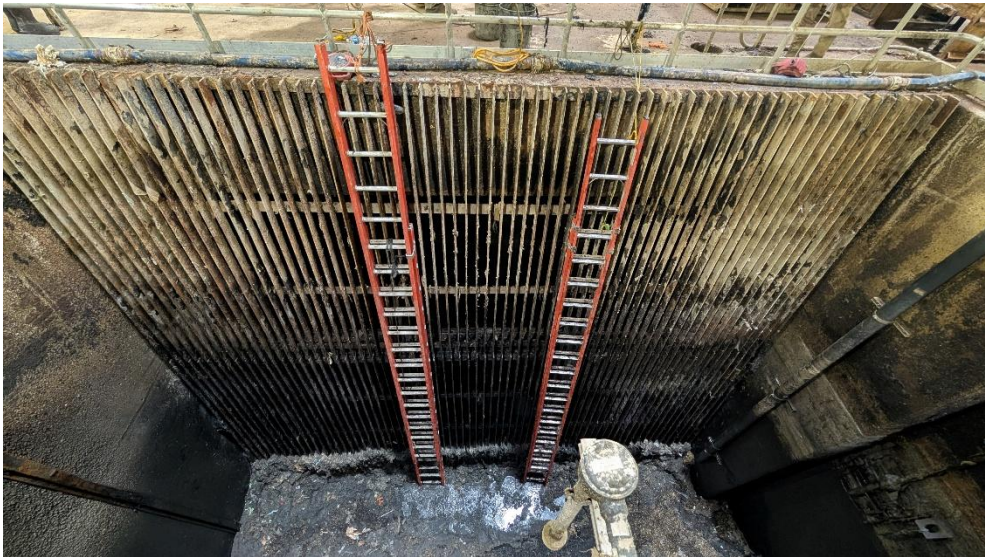
South side wetwell bar-screens after cleaning
