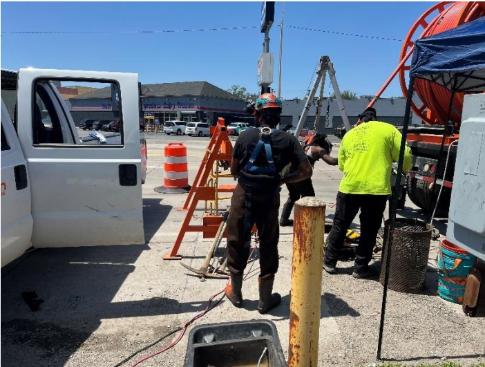
Entering PCI-19 to place grit catchers and winch lift
