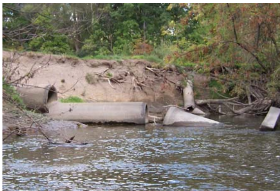
Eroded storm pipe, headwall, and bank at Beech Woods Park
