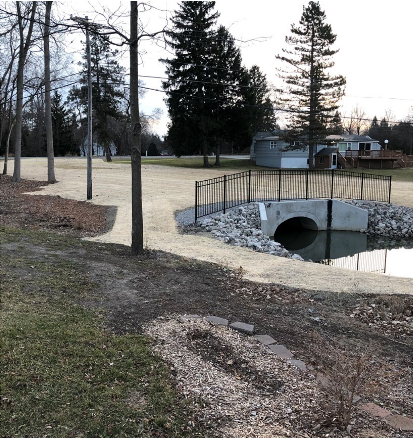
Photo 1: Completed headwall, fence, and restoration.
