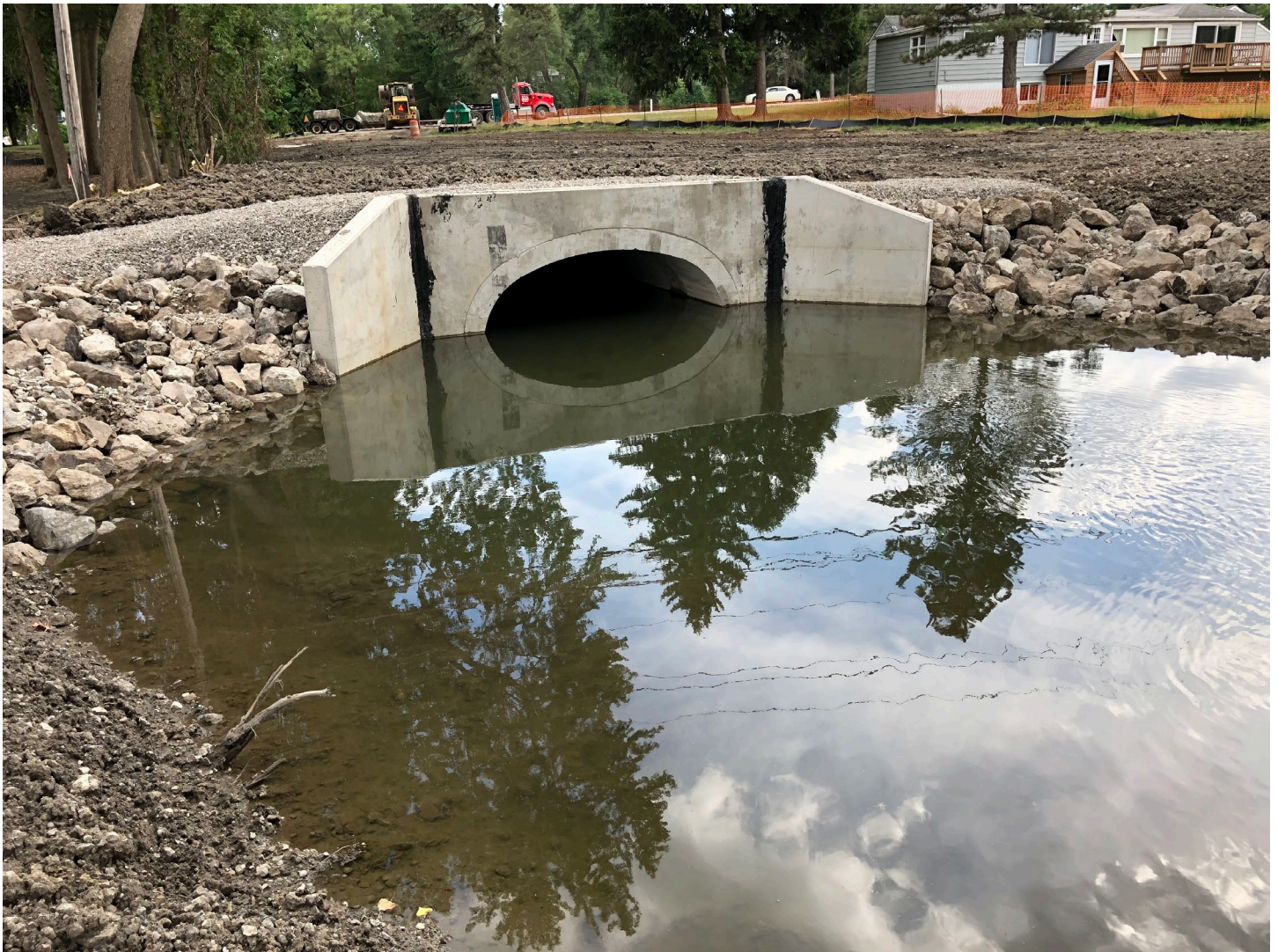
Completed Headwall
