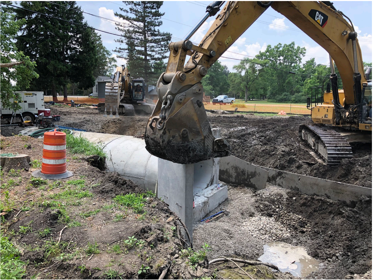
Installation of Headwall
