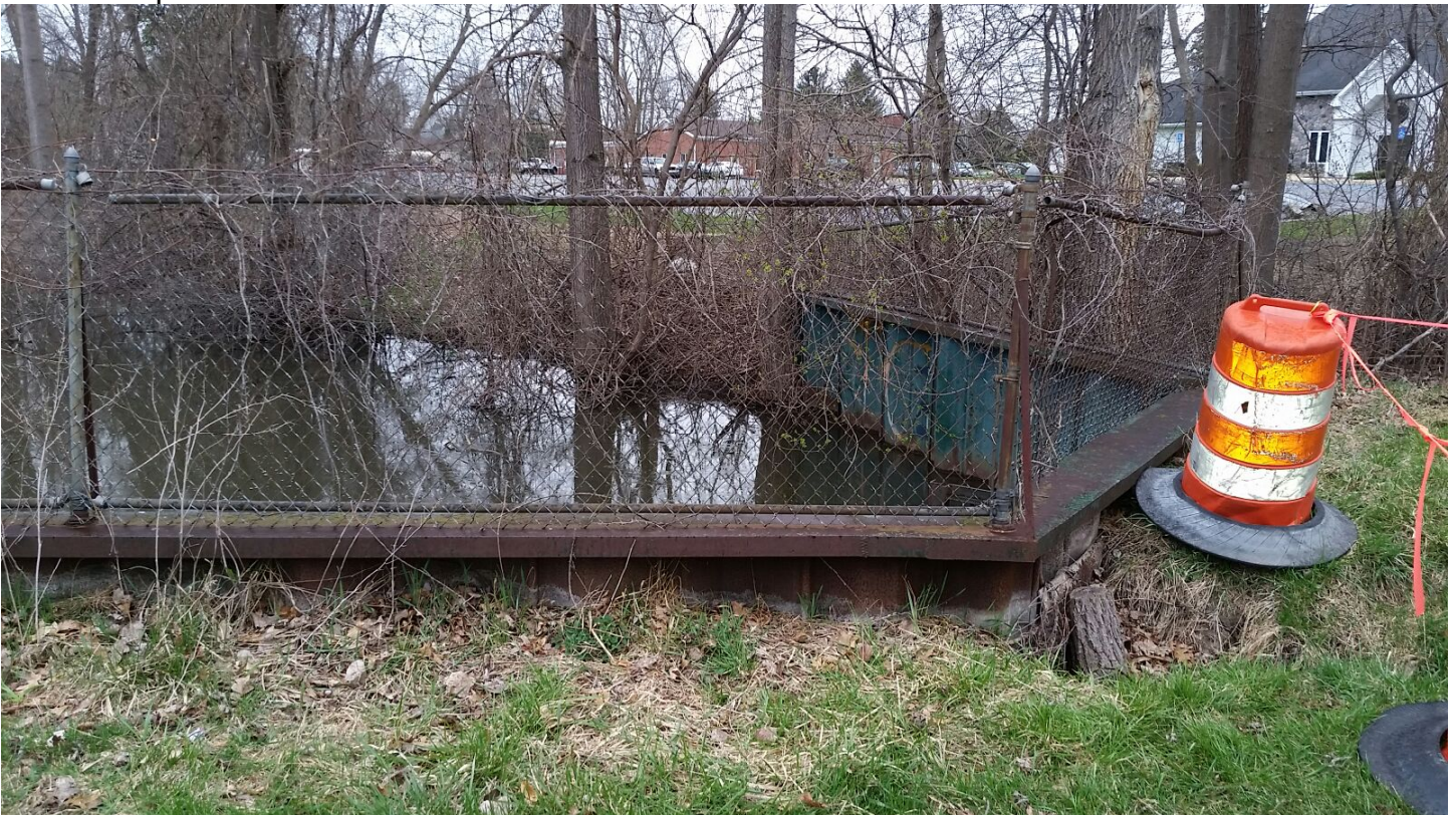
Metal Sheetpile Headwall
