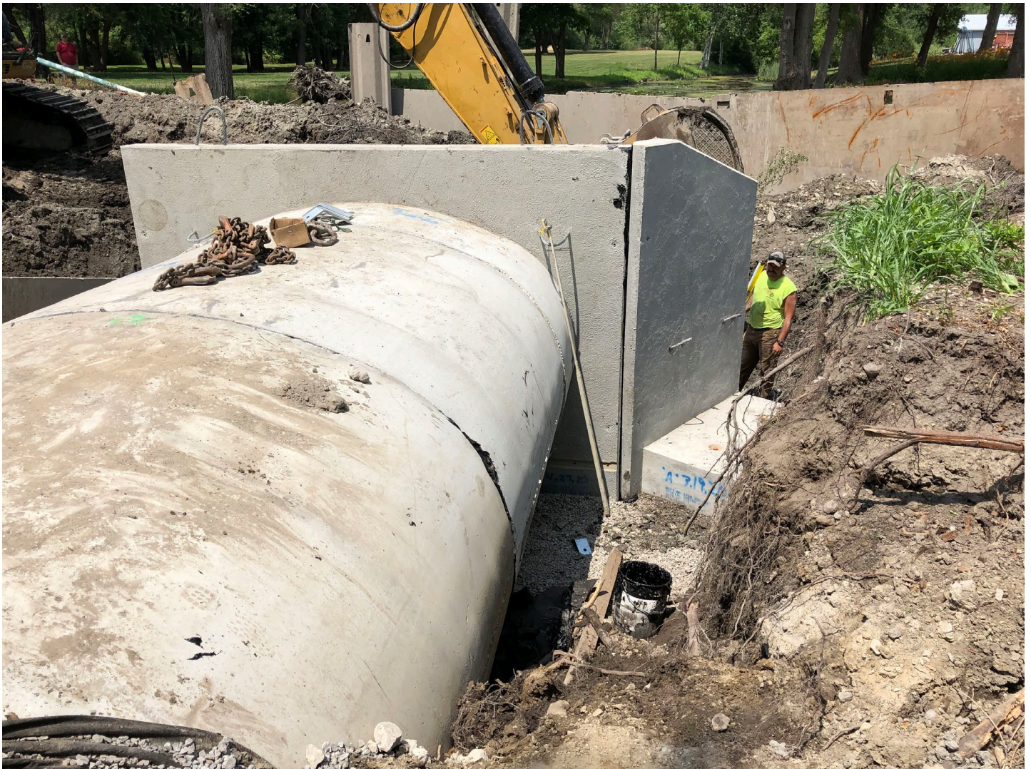
View of Headwall From Downstream Pipe
