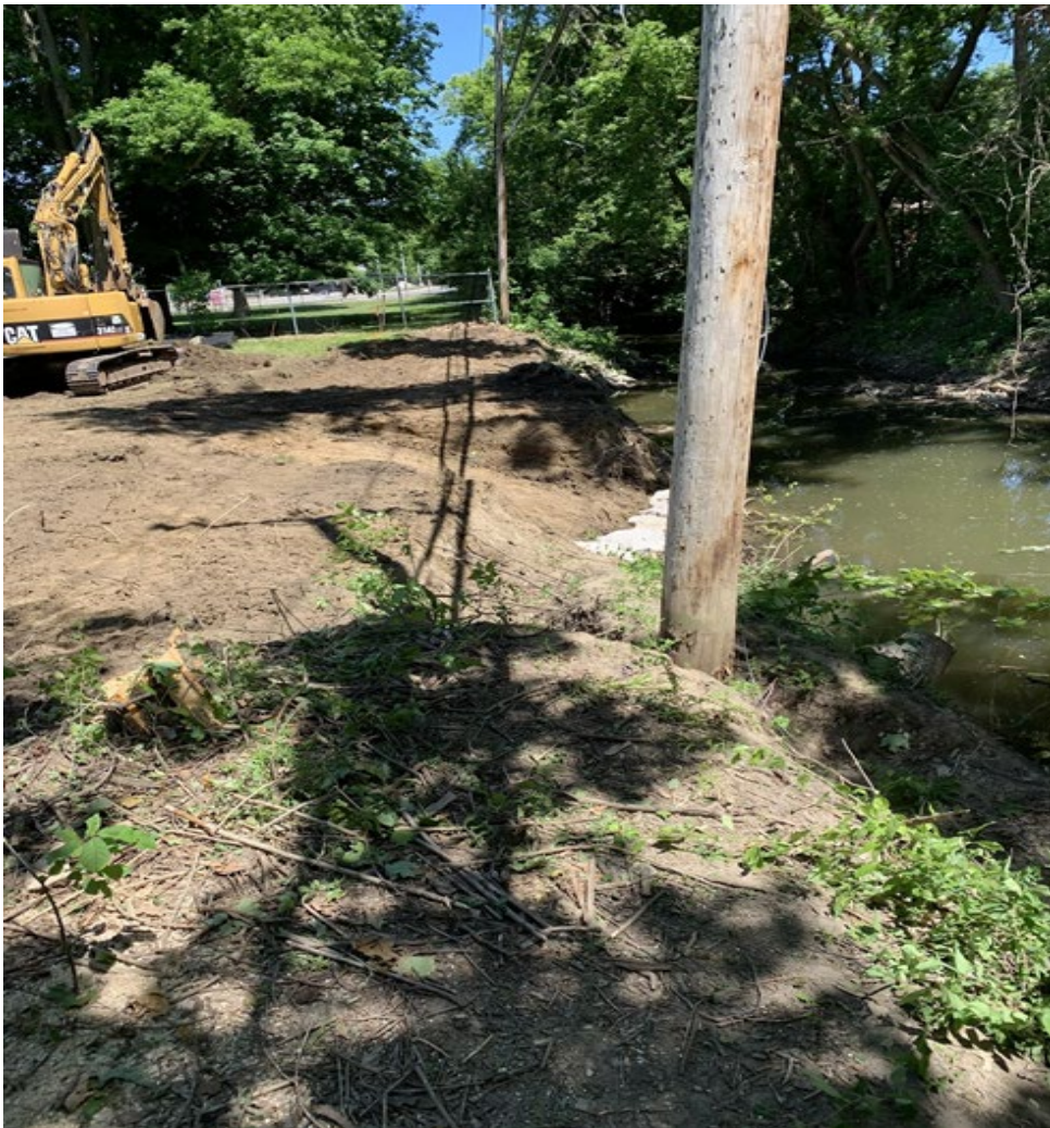
Eroded bank at power pole (north bank)
