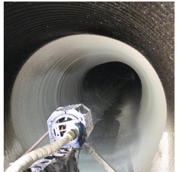
Figure 8: Spray application of a geopolymer lining
