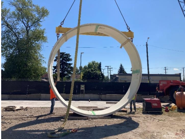
Topside staging of Channeline pipe segment
