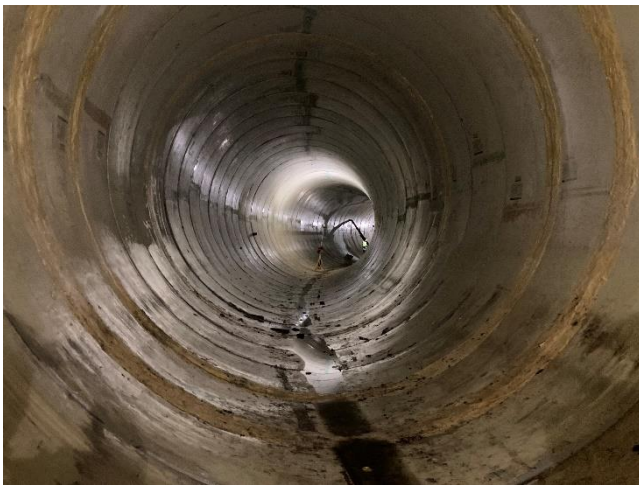
Looking downstream at Channeline segments installed in curve
