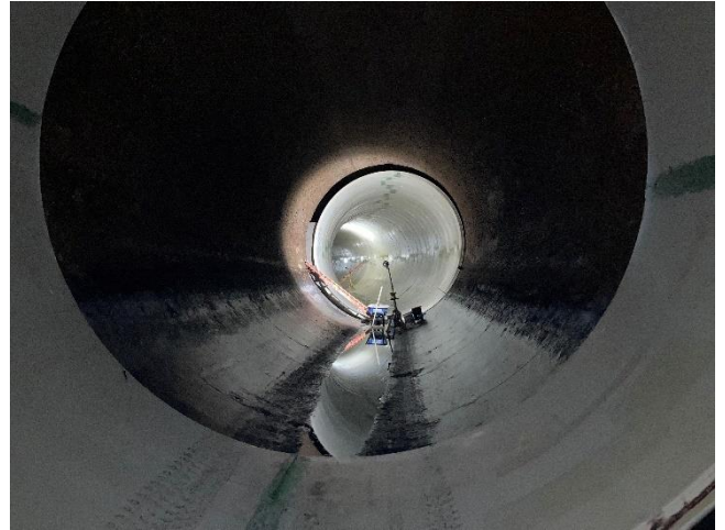
Looking upstream at progress of Channeline installation through September 2022
