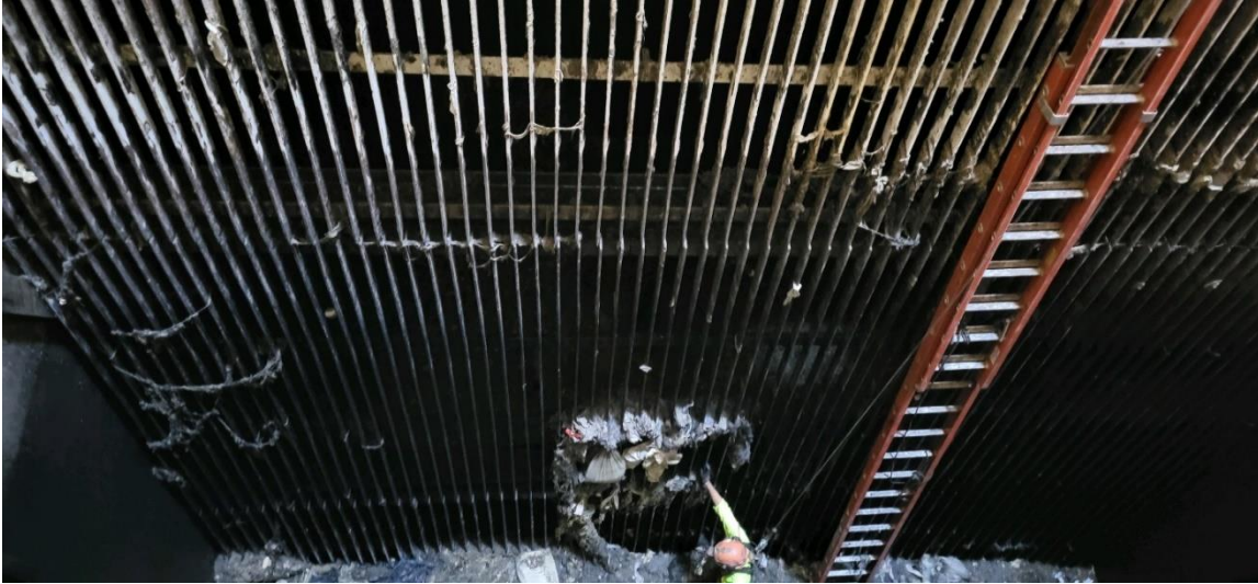
Bar screen cleaning in progress
