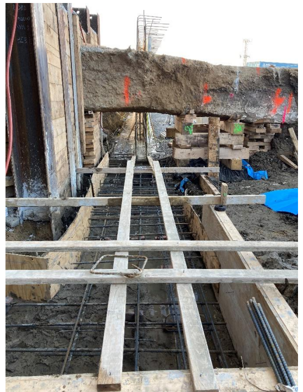
Ongoing work to support duct bank to transformer bay in December.
