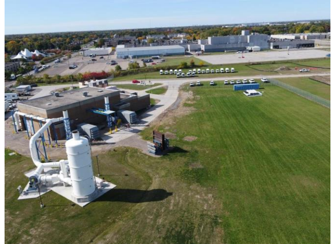
Biotrickling filter in full operational mode
