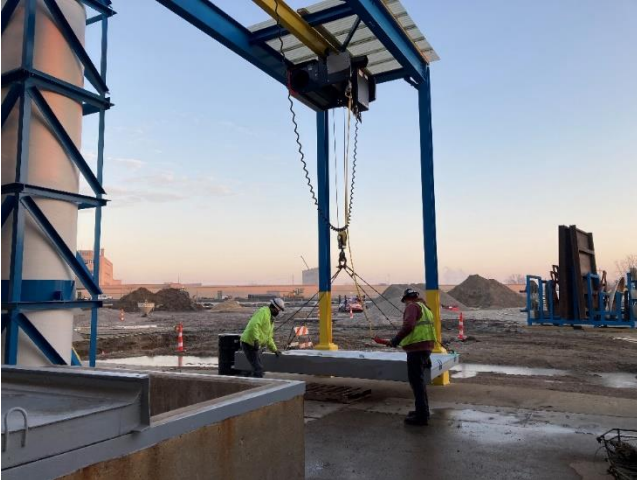
Walsh/DeCal Mechanical removing wet well hatch covers for planned inspection prior to knife gate installation.
