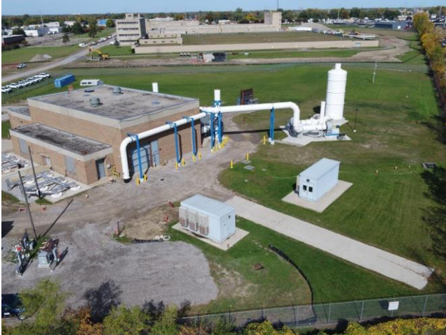
Biotrickling filter in full operational mode
