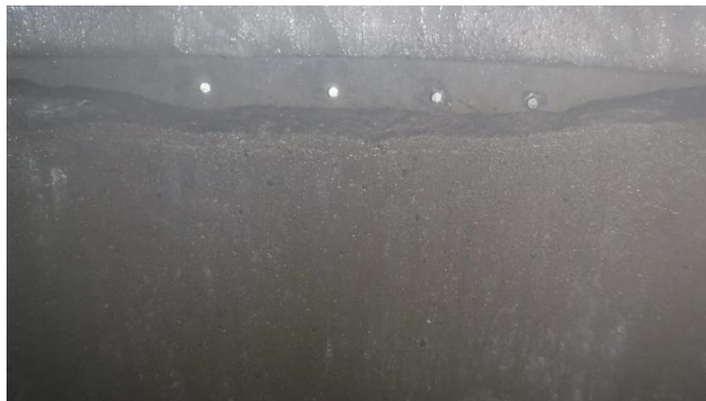
Example of deep concrete repair anchoring
