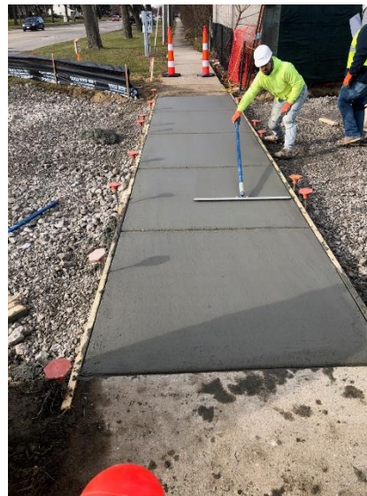
Finishing concrete for sidewalk across entry
