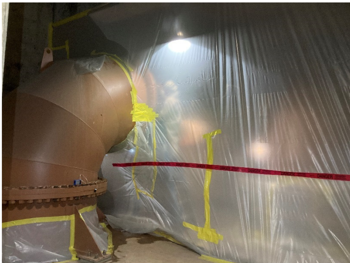
External Coating of discharge piping in progress
