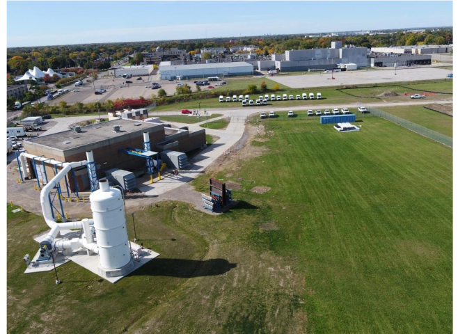
Biotrickling filter in full operational mode
