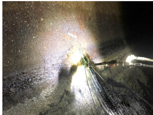
Chemical grouting in PCI-10A
