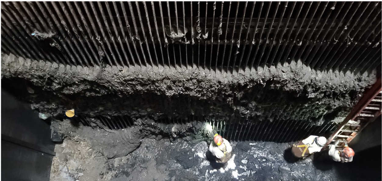
Wet Well cleaning in progress
