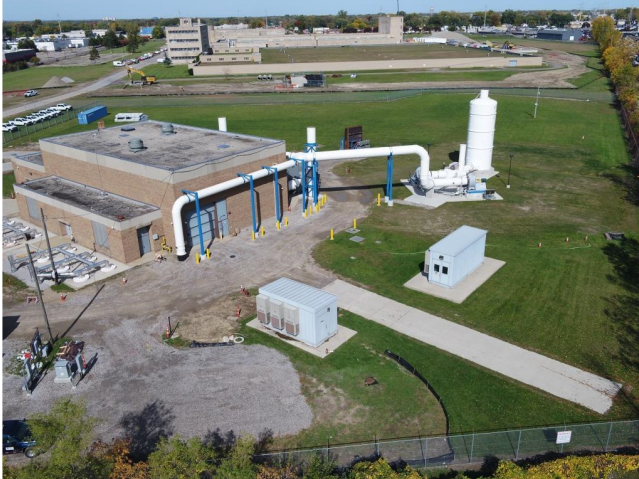
Biotrickling filter in full operational mode
