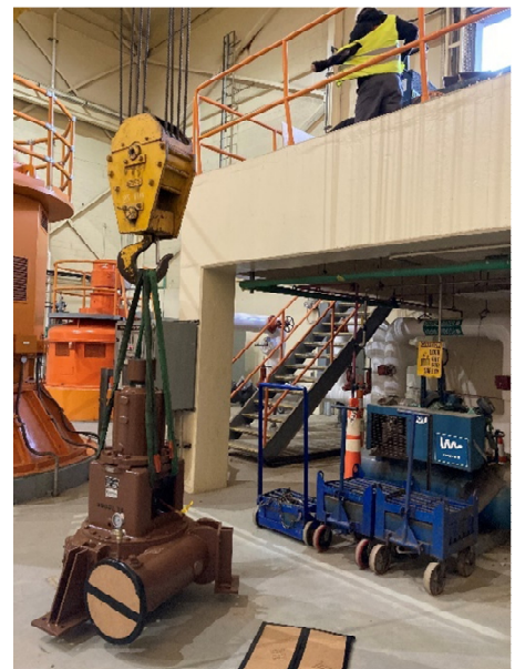
Delivery of new dewatering pump
