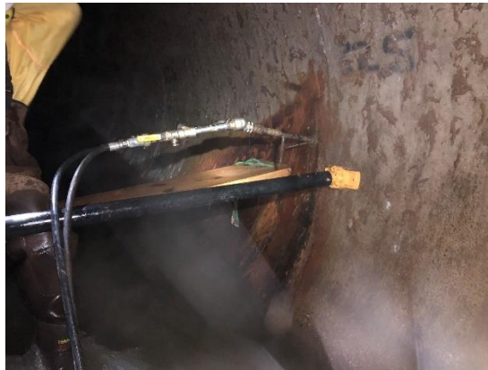
Chemical grouting in PCI-10
