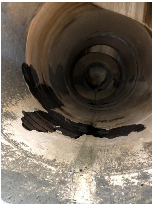
West manifold Thnemec Coating Deterioration
