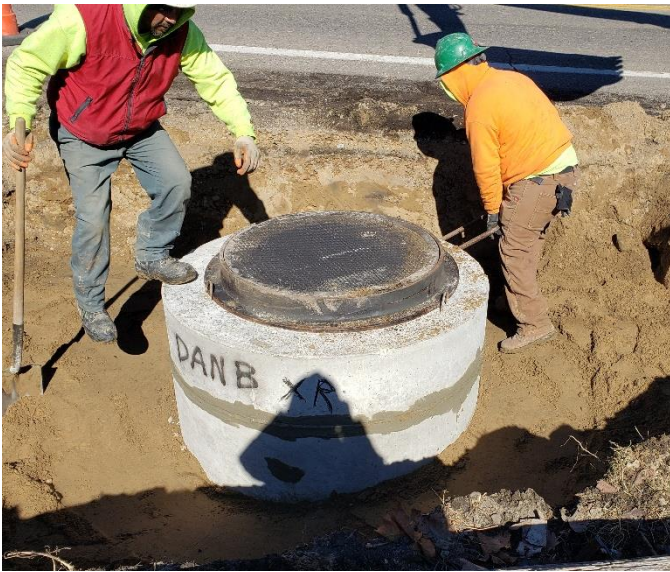
Manhole modifications in progress
