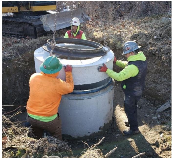
Manhole modifications in progress
