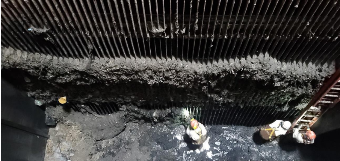
Wet Well cleaning in progress
