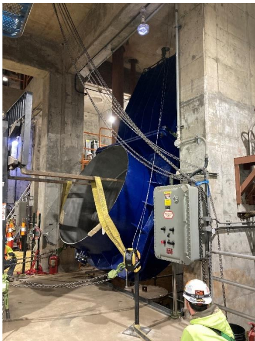
Installation of Knife Gate Valve 3 in March, 2021
