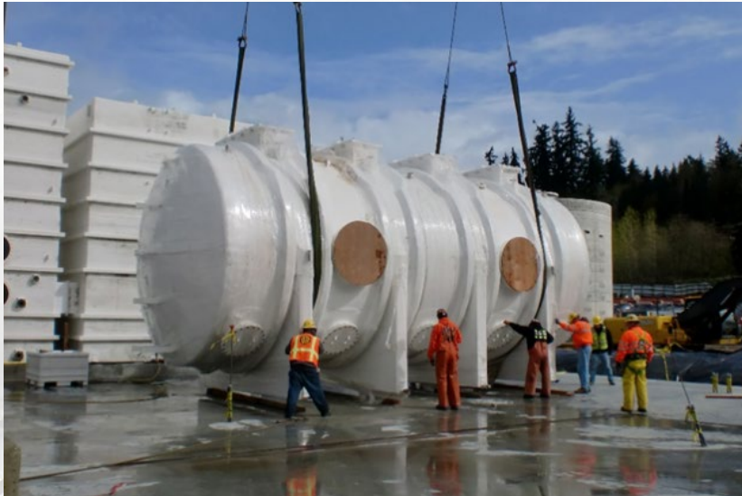
Carbon adsorption vessel
