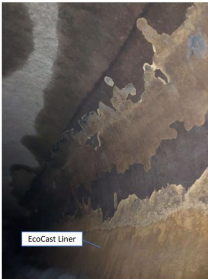
Upper 110' of PCI-4 lining peeling and failing in Feb 2021
