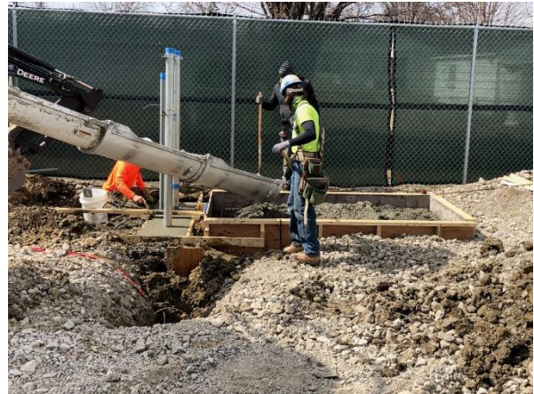
Pouring slab for control cabinet at CS-9 on March 16 th , 2021
