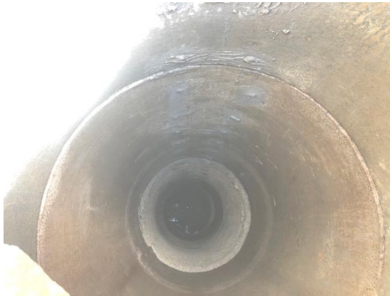
Manhole steps removed at Location #2
