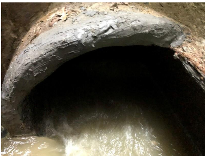
Spalling repairs in PCI-11
