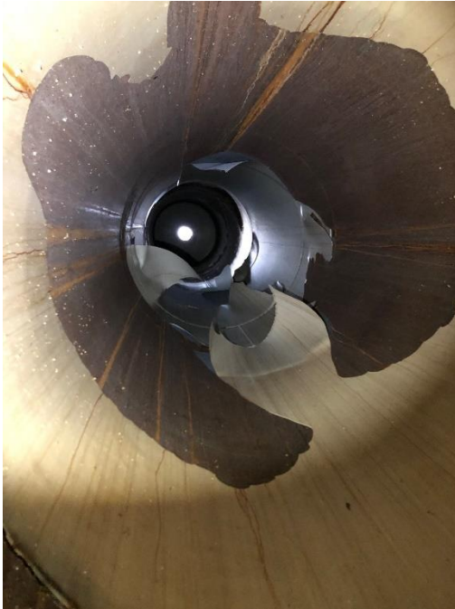
West manifold Riser, Tnemec Coating Deterioration
