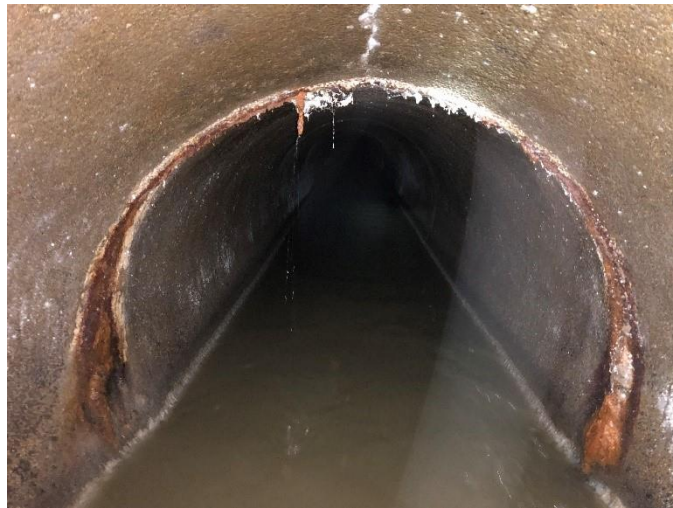
Running infiltration prior to chemical grouting in PCI-11
