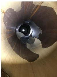
West manifold Riser, Tnemec Coating
