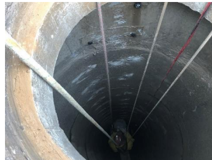
Typical patching of removed manhole steps
