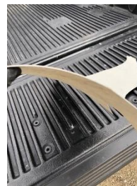
West Manifold Close-up of Peeled Coating
