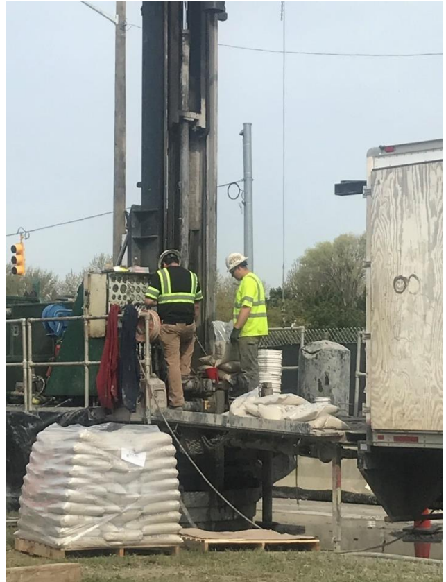
Contractor Installing dewatering well on 4/27/2021
