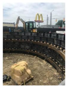
Installation of liner plate TERS underway on May 24
