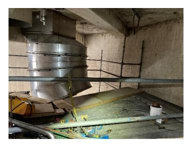
Wet well make up air unit duct line below deck
