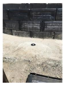
Inclinometer installed for geotechnical monitoring of shaft construction
