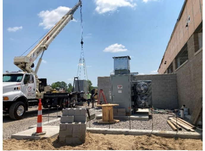
Placement of HVL near new Transformer 3
