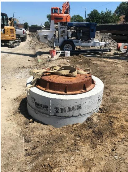
New manhole structure placed June 9, 2021
