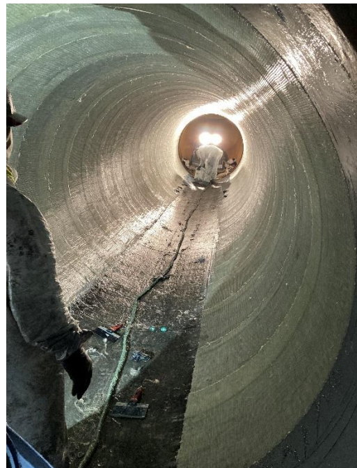
Pump #1 discharge piping – after first layer of QuakeWrap lining
