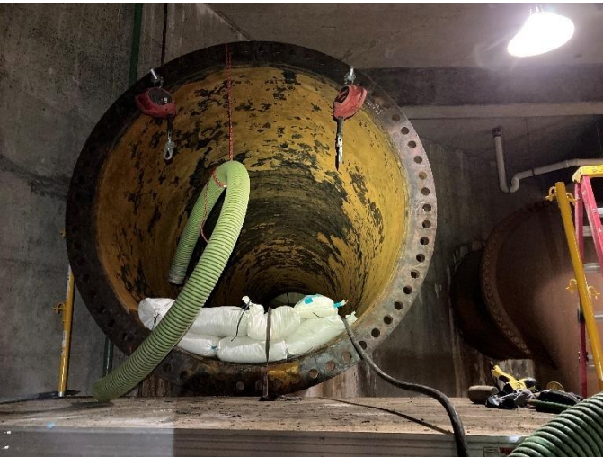
Pump #1 discharge piping – prior to lining
