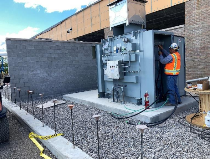
Landing new Transformer 3
