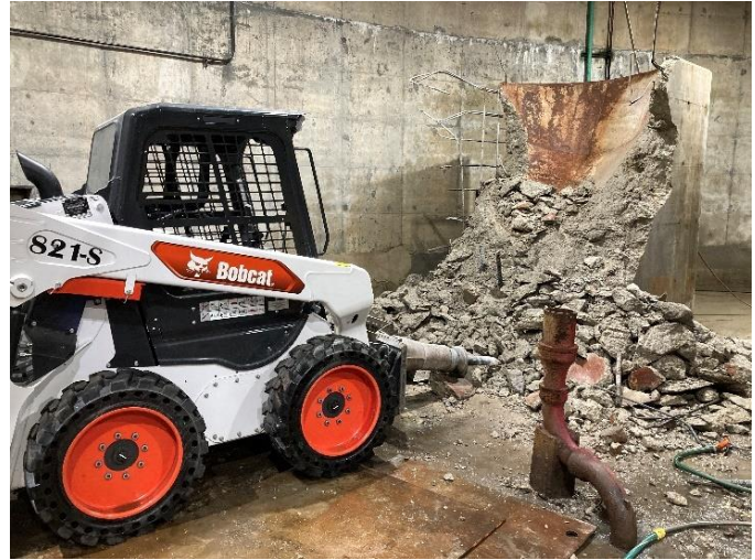
Demolition of Pump #1 discharge piping thrust block
