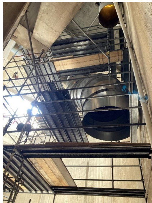
Wet well make up air unit stainless steel duct elbows below deck
