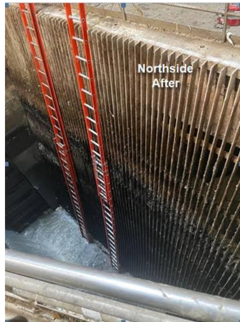
North side of wet well before and after recent cleaning efforts
