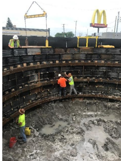
Crews working to construct liner-plate TERS in early June, 2021
