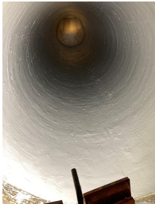
Completing QuakeWrap lining of P1
