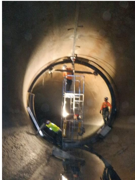
Crews working to install internal ribs on July 22, 2021
