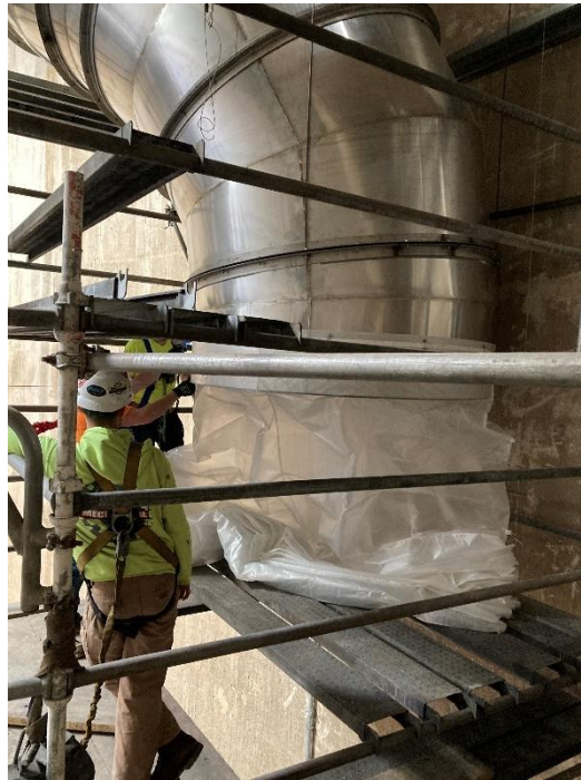
Wet well make up air unit stainless steel duct elbows below deck (now complete)
