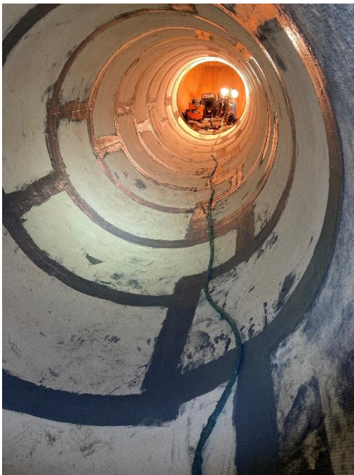
Completing QuakeWrap lining of P1
