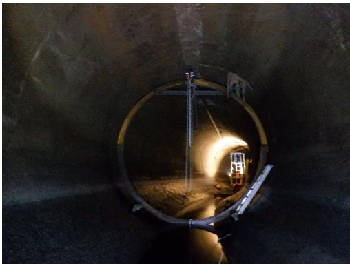
Internal rib and monorail installation on July 21, 2021
