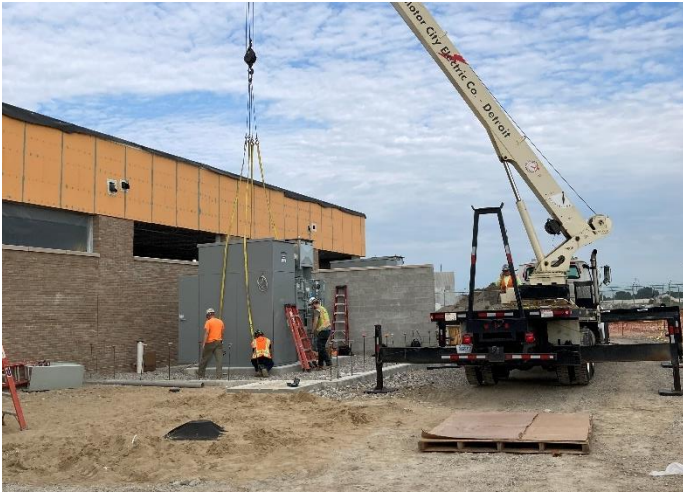
Placing components for Transformer #4
