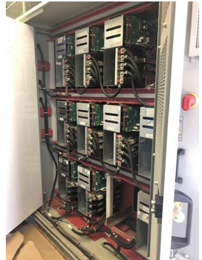
Sanitary Pump #2 VFD power cells
