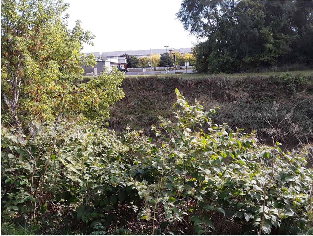
Photo 3: Looking at north (left) bank upstream of Van Dyke Ave. Steep banks, bare soil near surface indicates slope failure. (Area 3)
