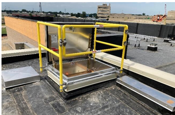
Safety rails at replacement roof hatch on August 18, 2021
