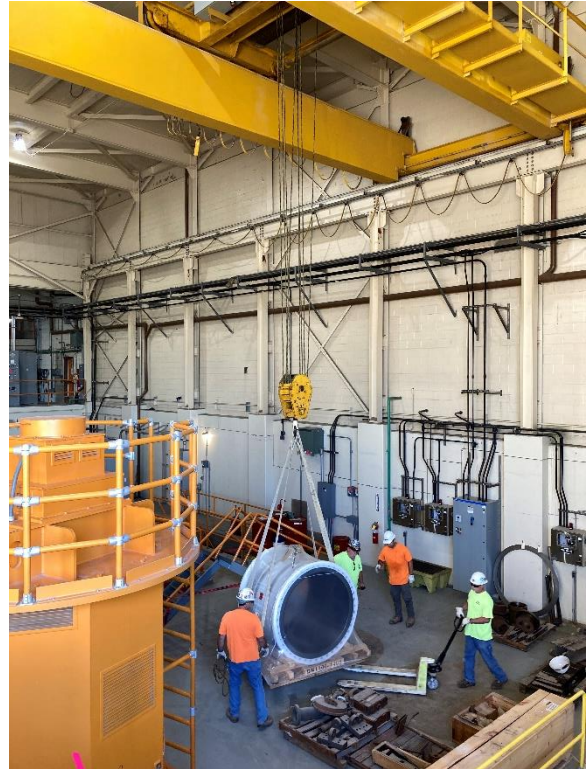
P1 Mag Meter installation on August 20, 2021
