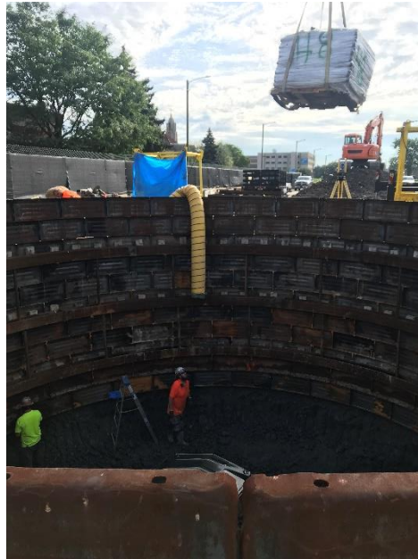
Marra bringing additional liner plate into shaft for ongoing construction of TERS on August 25, 2021
