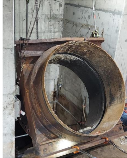
Removal of bonnet at Knife Gate #1 in early October, 2021
