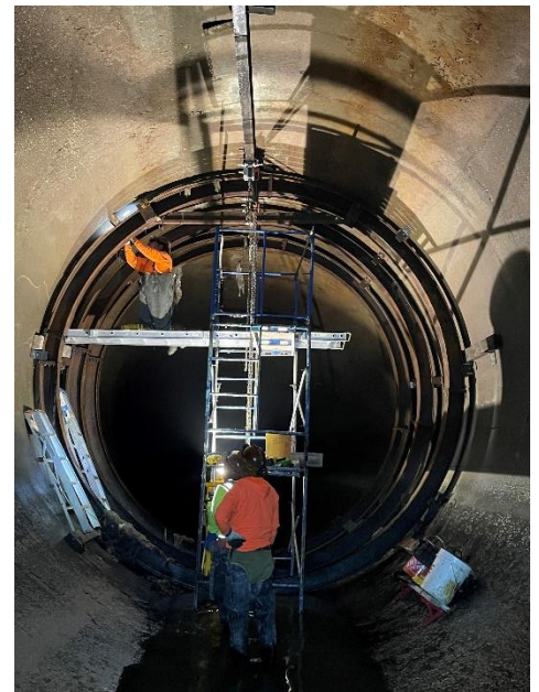
Marra continuing installation of in-sewer support on September 29,
