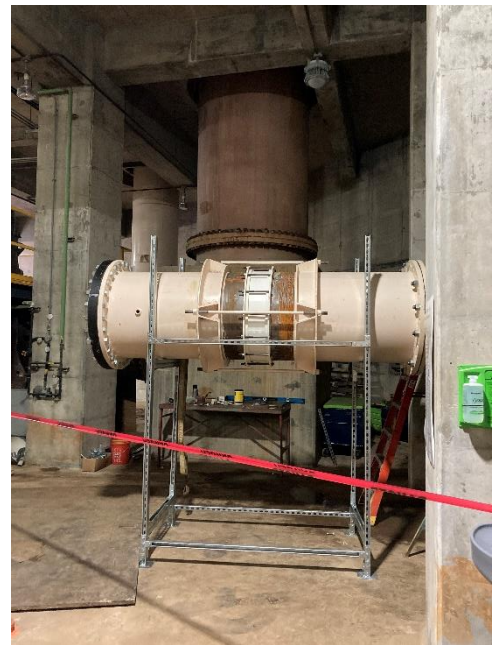
New Pump #3 pipe and elbow build
