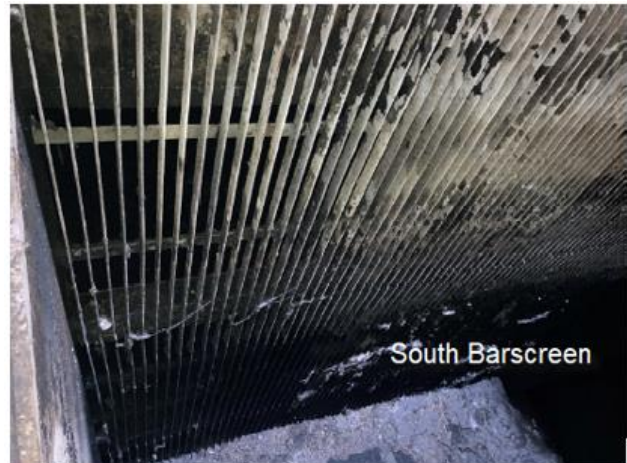
Status of bar-screens during sediment inspection
