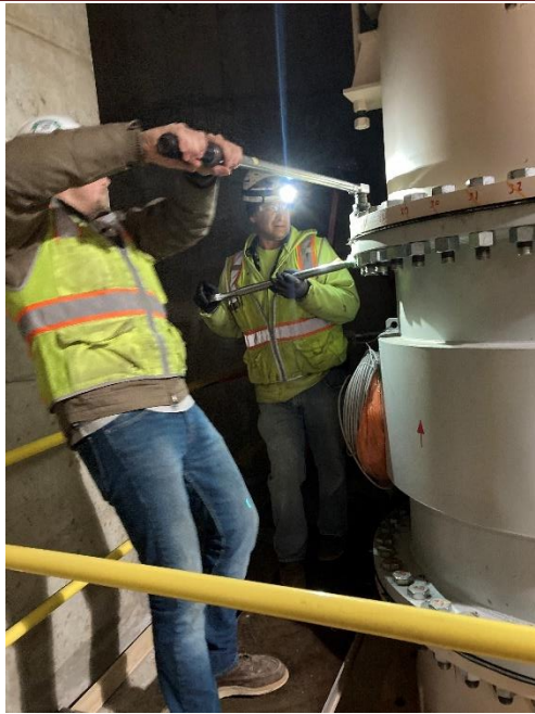
Adjustments to flow meter flange bolt at Pump #3 discharge pipe
