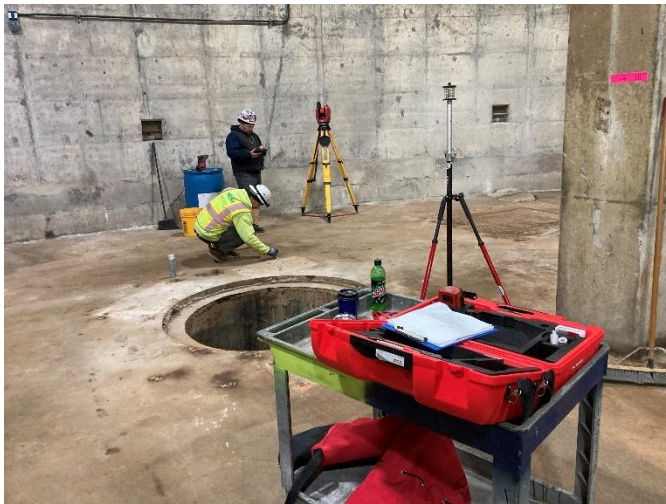
Lay-out of alignment for Pump #1
