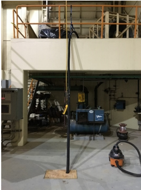
Preparation for temporary water supply during upcoming water shutdown.
