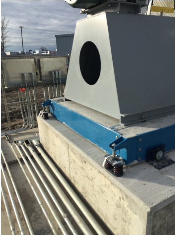
Installation of the odor control fans on vibration control bases and additional installation of biotrickling filter electrical conduit.
