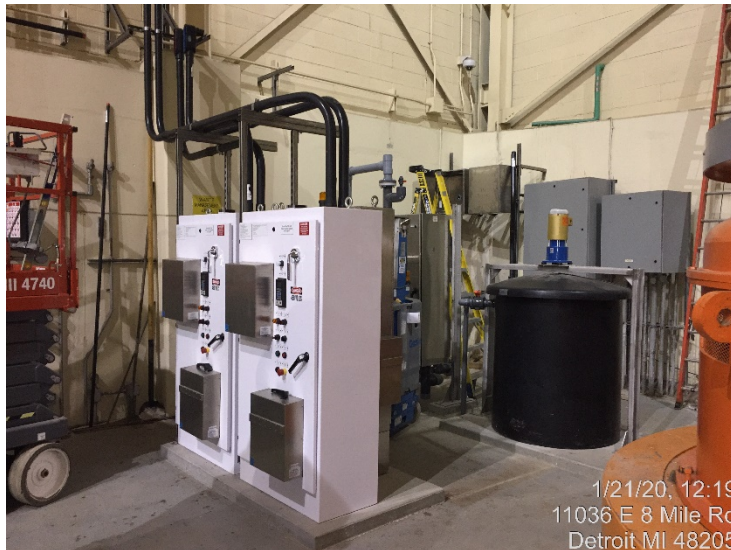
Installation of BioAir VFD cabinets and control panel; Additional water and drain pipe installation along the biotrickling filter vessel.
