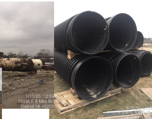
Demolition of existing duct work on the west side of the wet well; HDPE and FRP duct work arrived on site ready for installation.
