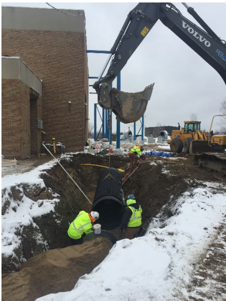
HDPE duct work installation ongoing; HDPE duct penetration into the gate house and backfill operations.
