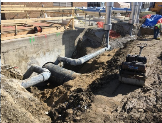
HDPE duct work installation ongoing; HDPE duct penetration into the gate house and backfill operations.
