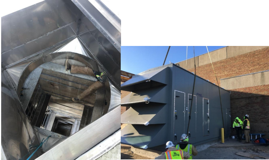
Installation of the wet well makeup air unit #1 and associated duct work in the wet well; along the biotrickling filter vessel.
