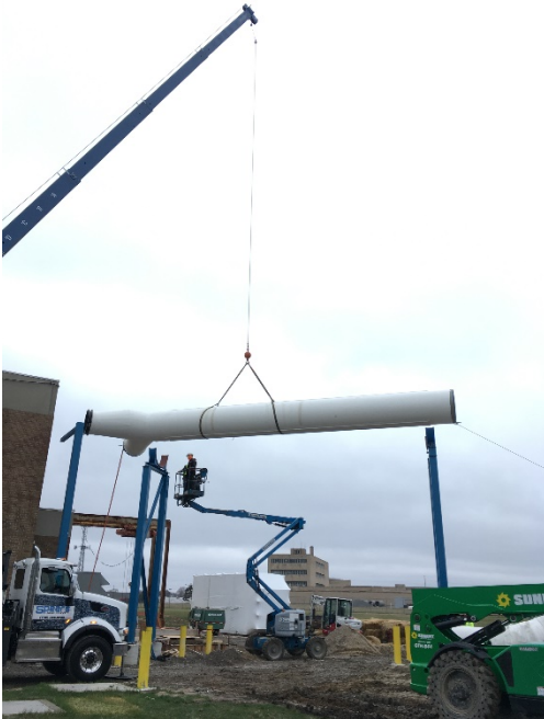
Installation of the FRP above ground duct sections and associated drain piping; along the biotrickling filter vessel.
