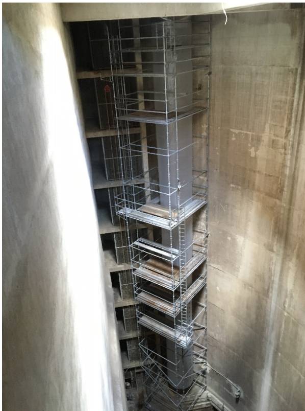
Installation of fabric duct on the west side of the wet well.
